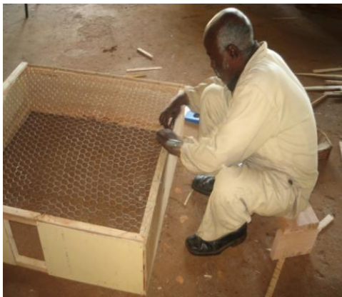
Photos 1-2 Construction of the hay-box brooding technology at JUCAVM
