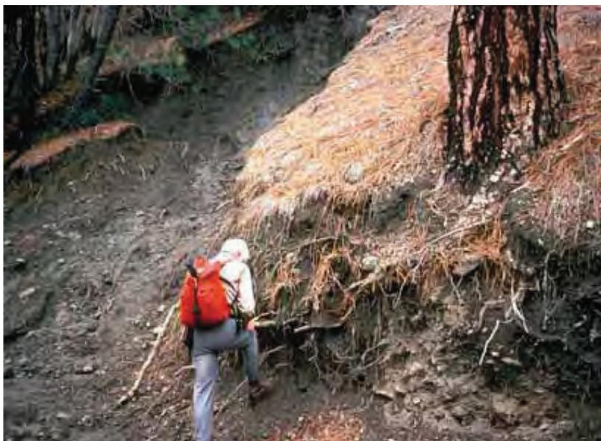
**Figure 2.4.** Ponderosa pine tree buttressing a slope above a forest road. The unprotected portion of road cut to the left has failed. Mendocino National Forest, California, 1978
