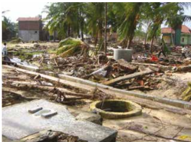
FIGURE 14 Toilet pits in close proximity to wells 14
