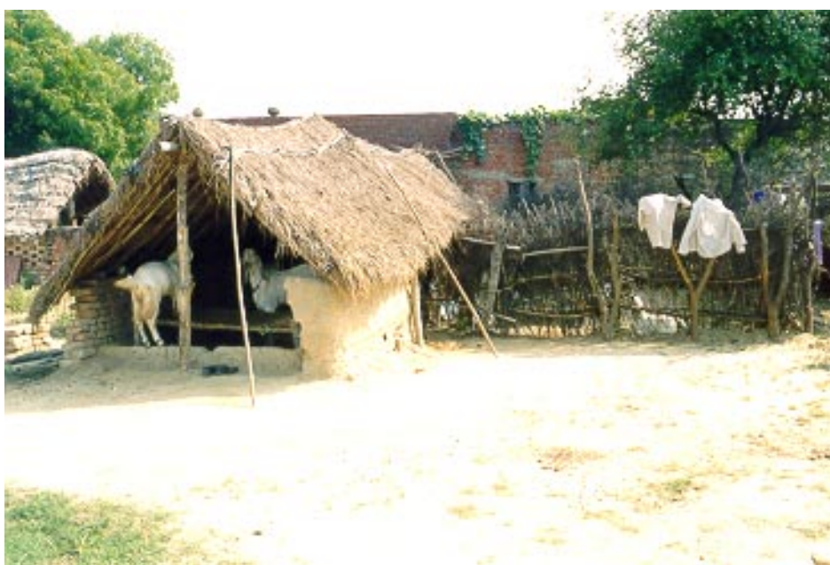
Figure 3. Covered accommodation are covered with thorny bushes and used for keeping the goats. Some times this structure may be made of mud or bricks.
