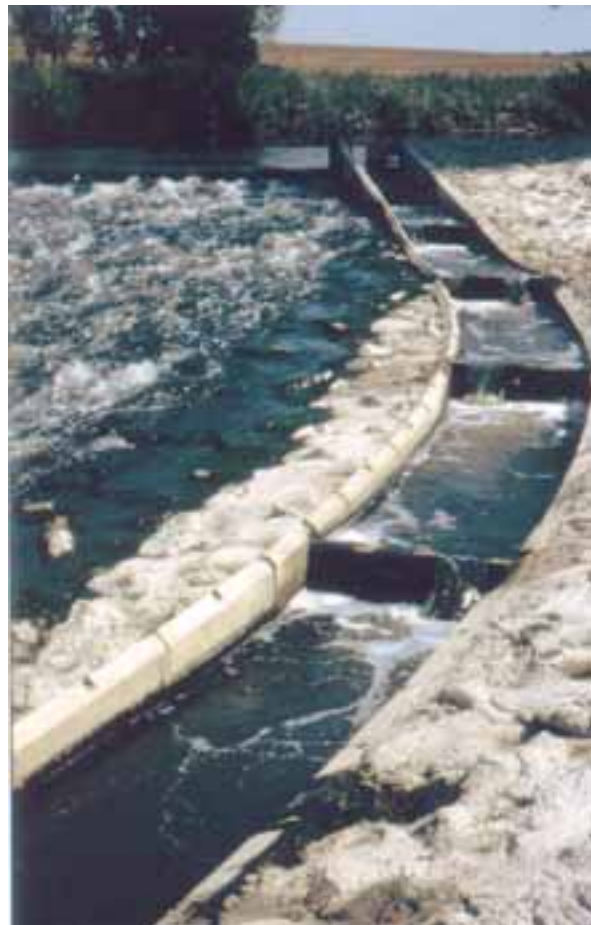
Fig. 5.13: Dahl pool pass in operation (view from tailwater)
