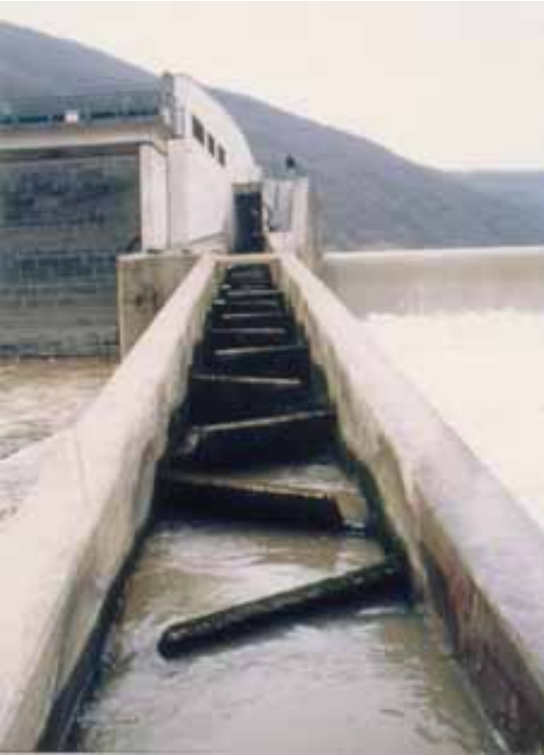
Fig. 5.7: Example of a rhomboid pass (Moselle weir Lehmen, view from tailwater)
