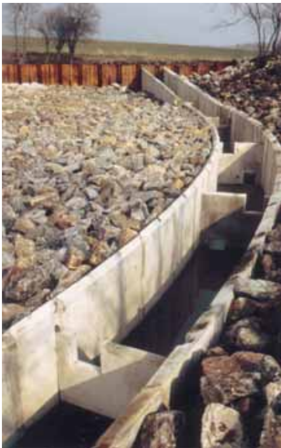
Fig. 5.12: Dahl pool pass (shortly before going into operation)
