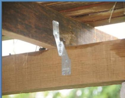
Between floor joists and floor beams
