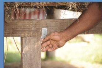
Between floor joists and floor beams
