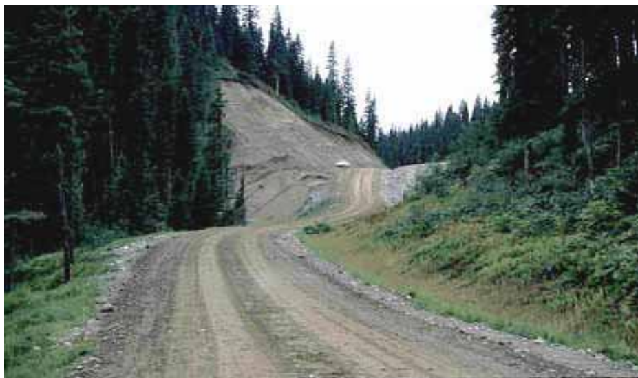
Stabilisation of the ditchline in erodible soils
