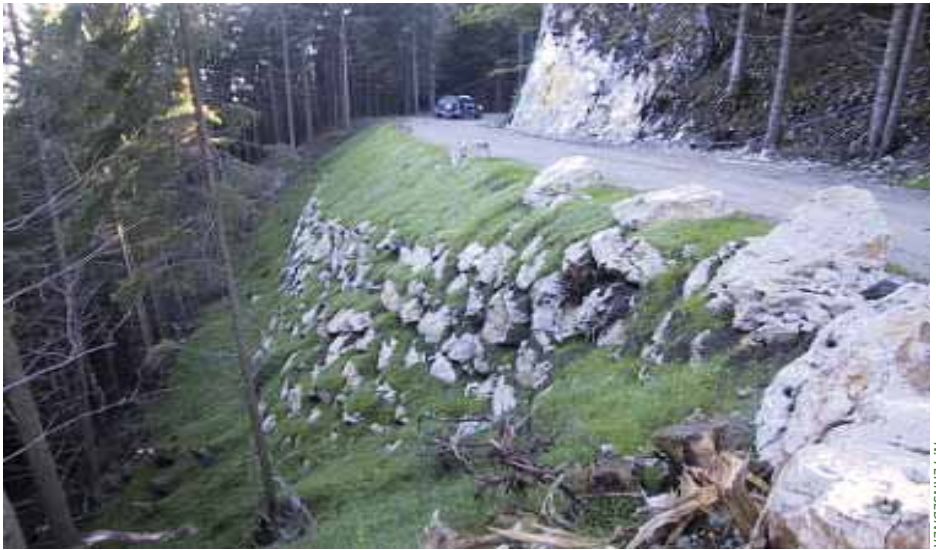
Dry stone retaining structure
