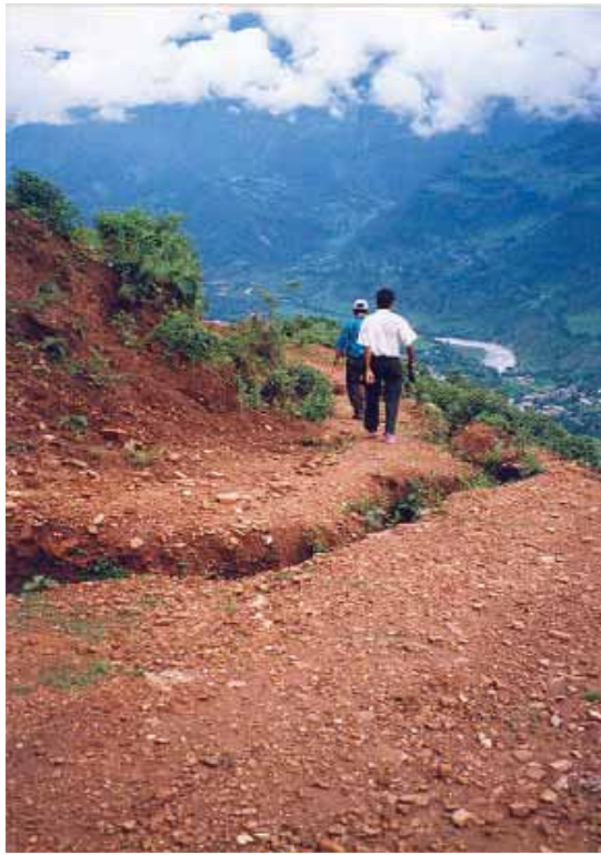
Potential consequences of inadequate drainage
