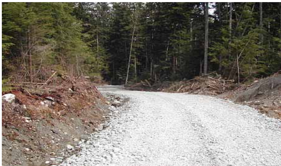
Placement of the base course aggregate to a designated thickness provides for an adequate load-spreading action
