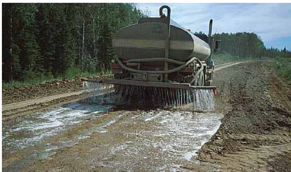
Application of a dust palliative
