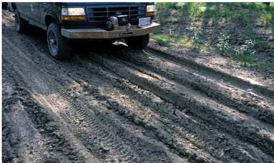
Cumulative effects of repeated loading
