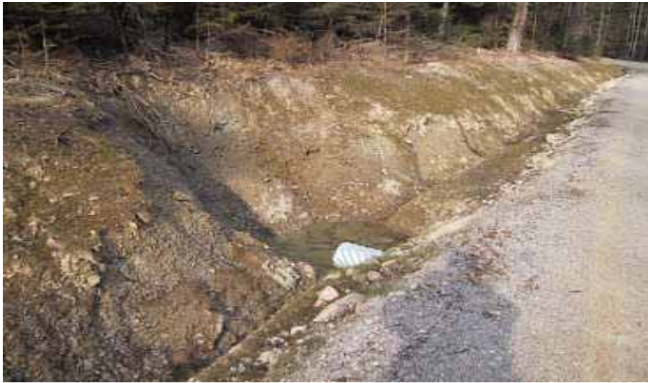
A corrugated metal pipe culvert, with ditch block at the culvert inlet
