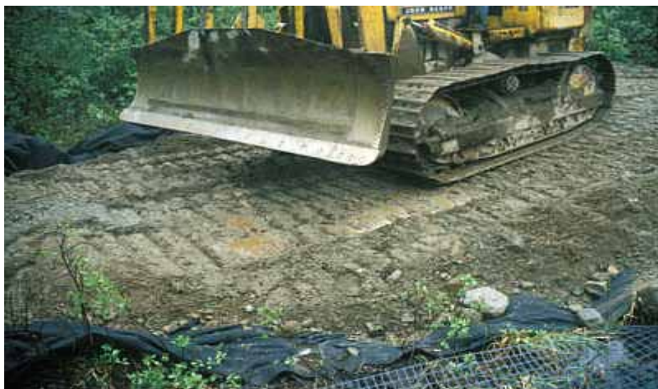
Spreading gravel over a geotextile, with a geogrid evident in the foreground
