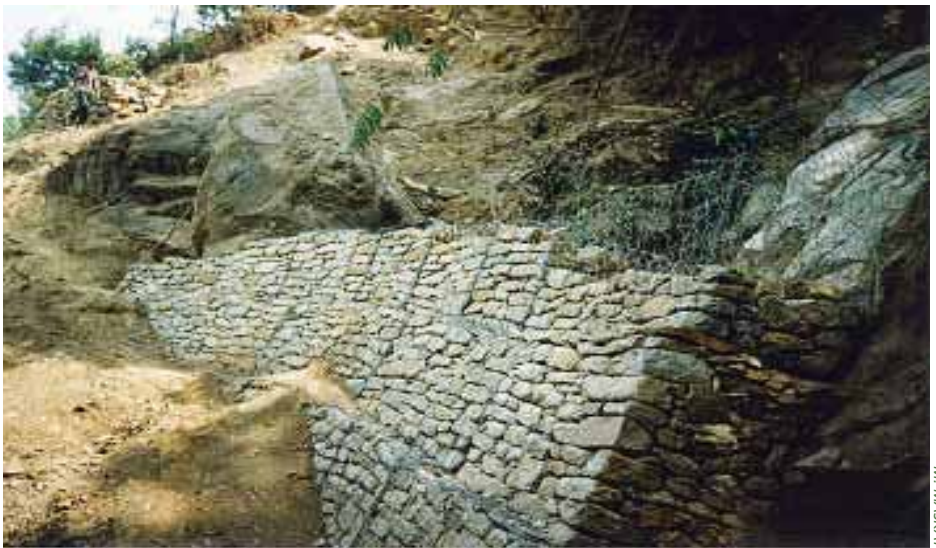
Gabion retaining structure
