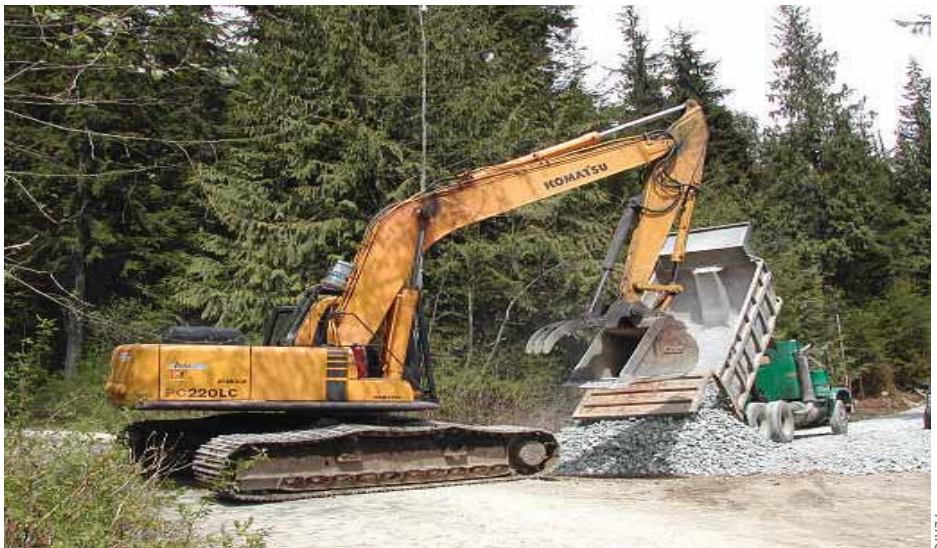
Resurfacing operation for road maintenance
