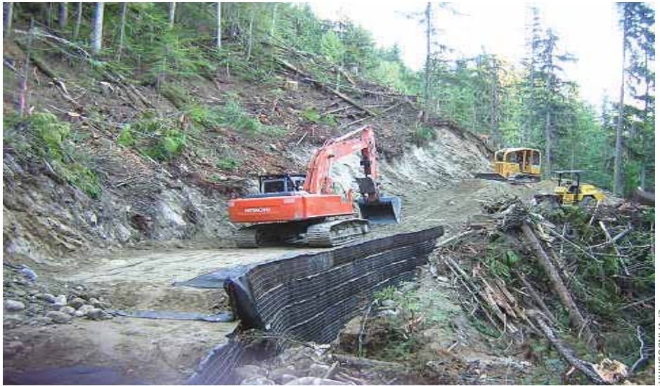
Geotextile reinforced soil wall
