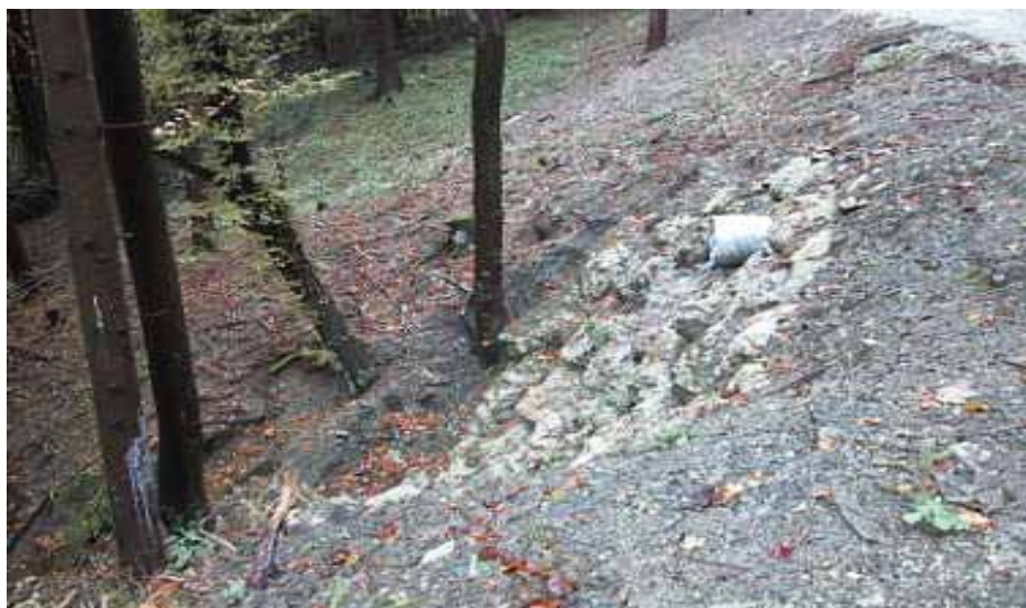
Scour protection at the culvert outlet
