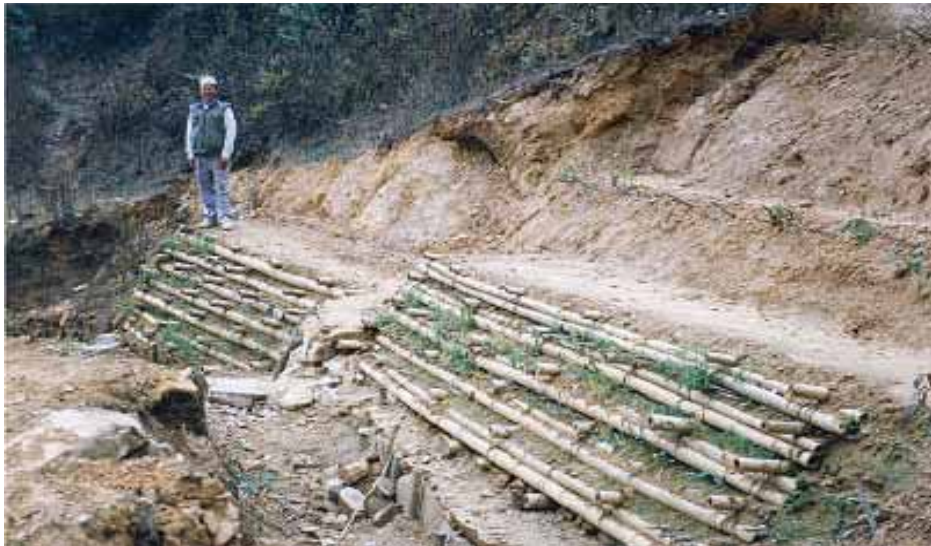
Planting of terraces for biotechnical stabilization
