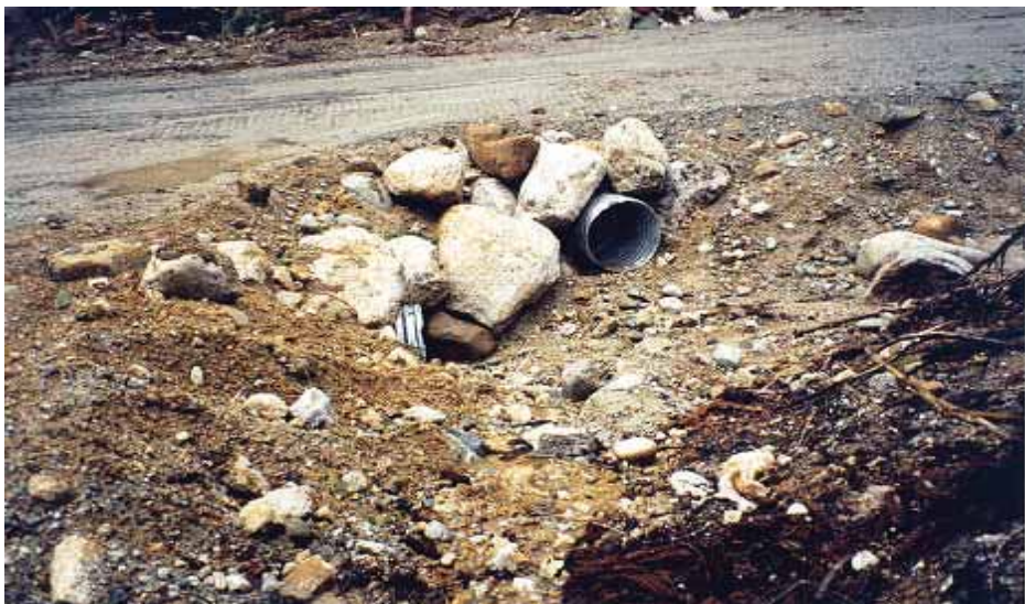
Angle or skew the alignment of the culvert to best direct flow to the inlet
