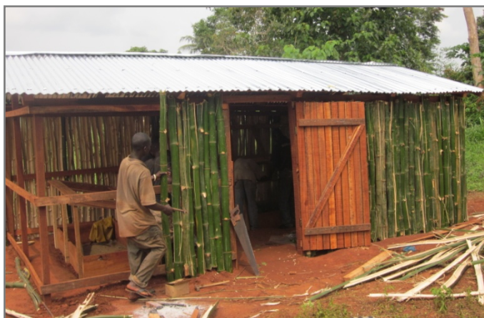
Picture 3: Covering the shelter's wall and constructing the propagator's rack, pilot site Mbaïki, Central African Republic (Photo: Bruno Bokoto de Semboli)
