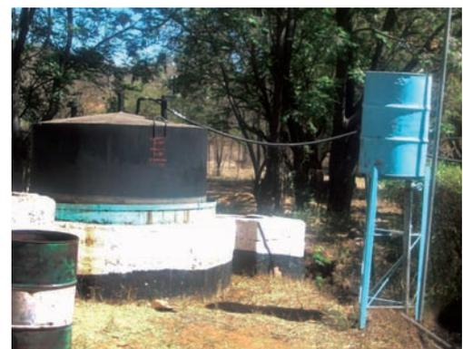
Gas collection tank resting on the concrete-built digester. Pipes / tubes at the top of the gas tank supply the house with methane gas, Botswana. (Reuben Sebegu)
