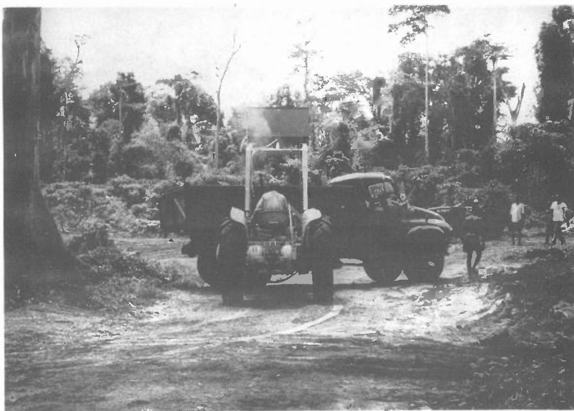
Gravel being loaded on to truck for gravelling main forest roads in a small forest operation company
