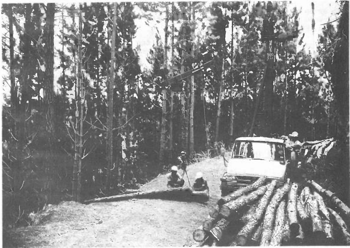
Mobile cable crane equipment extracting logs in thinning operations
