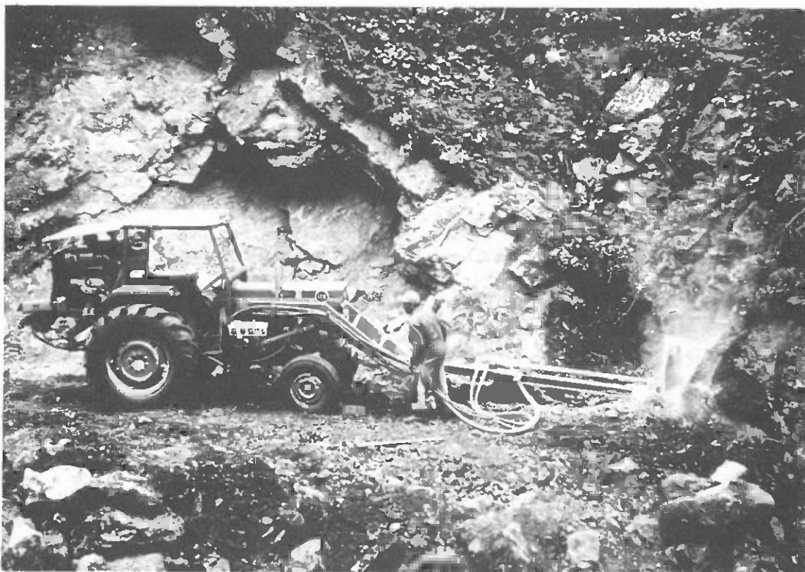
Mechanized drilling to speed up road construction in rocky mountainous terrain
