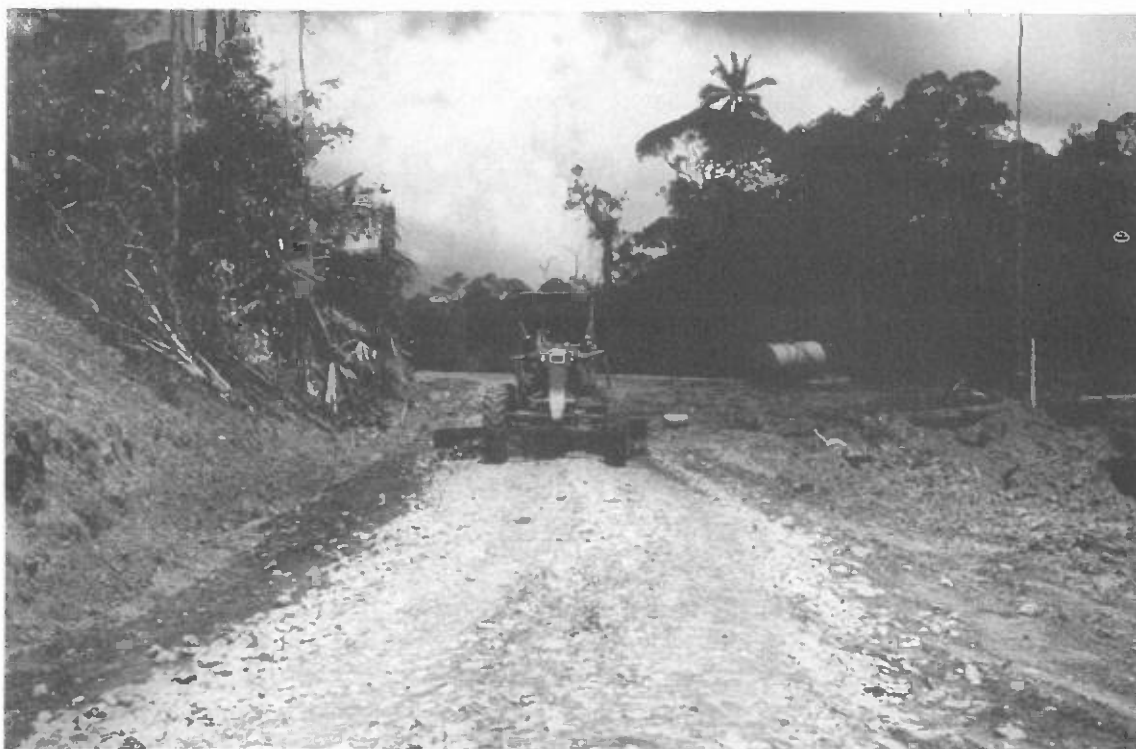
Motor grader reshaping a main forest road during road maintenance
