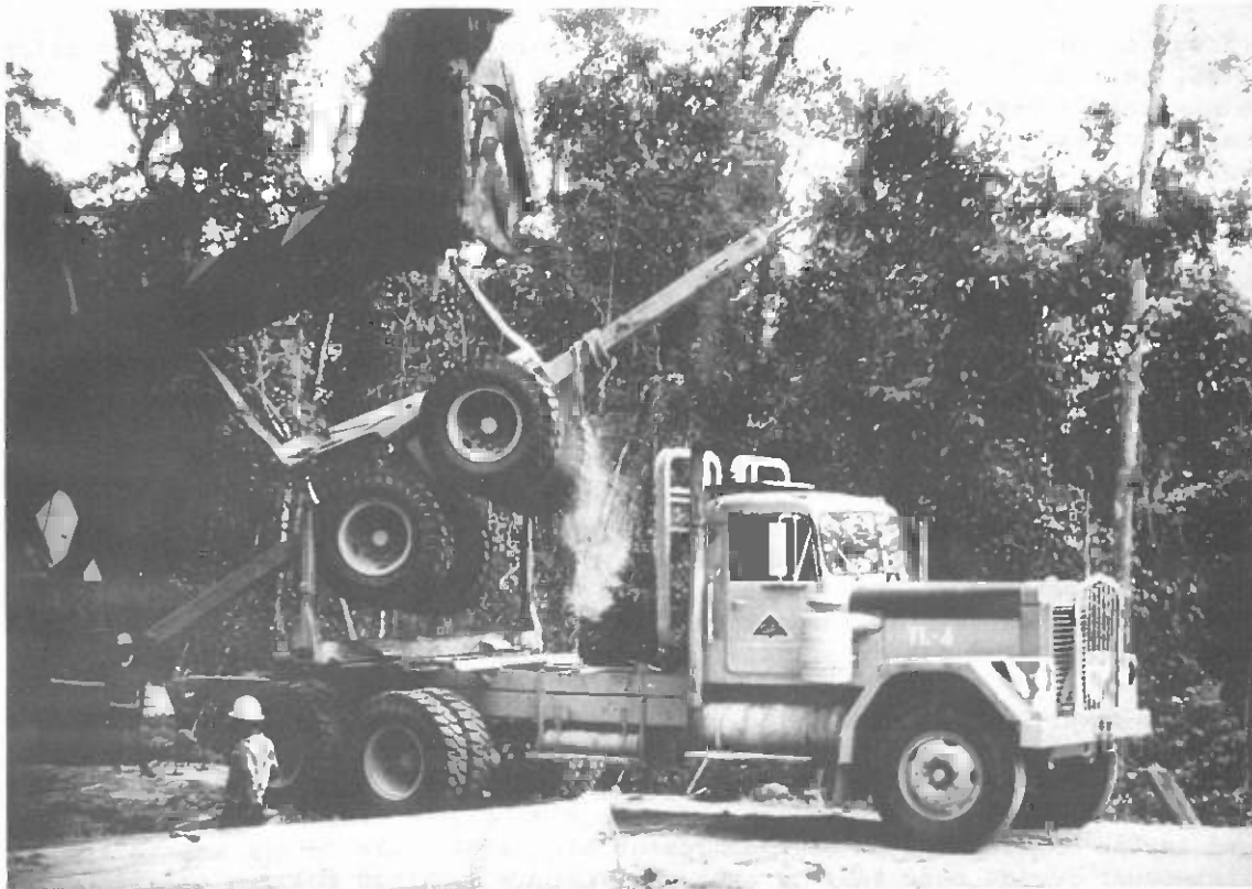
Unloading of tandem axle semi-trailer to be connected with truck head for log transport
