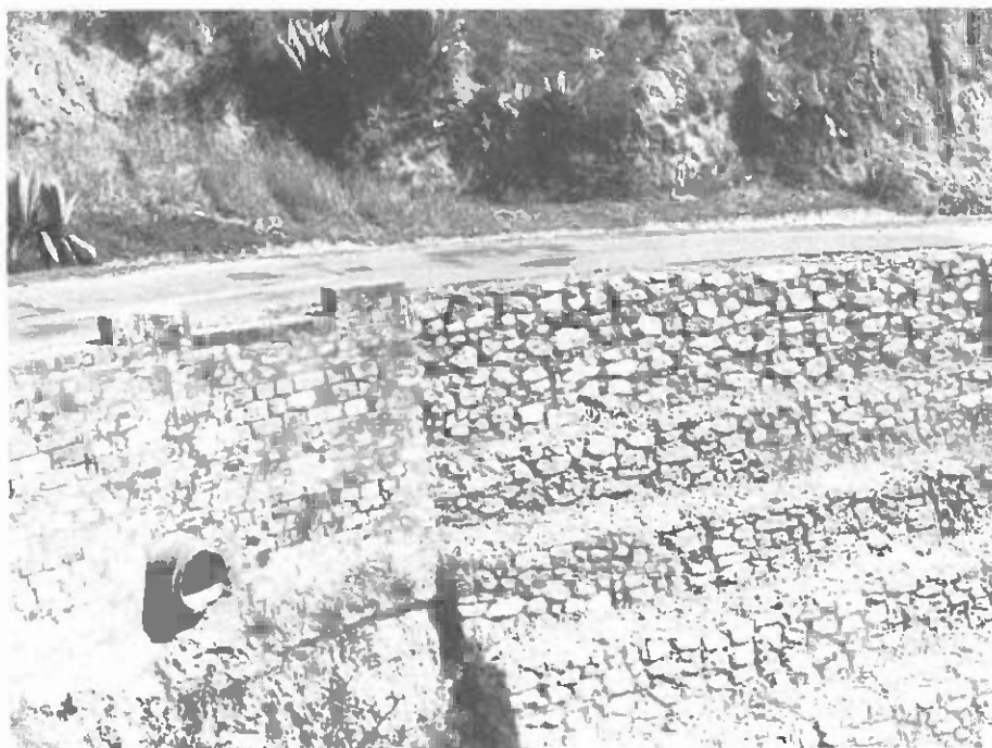
Destroyed retaining wall efficiently replaced by gabions (Photo: R. Heinrich)
