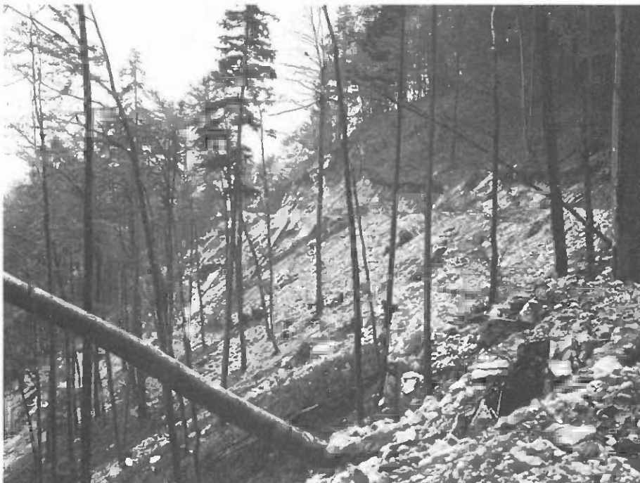
Blasted material deposited on a steep slope (Photo: M. Jedlitschka)
