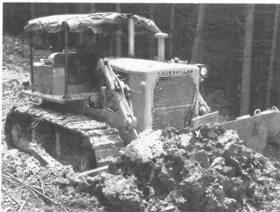
Heavy-duty tractor engaged in road formation work (Photo: O. Sedlak)
