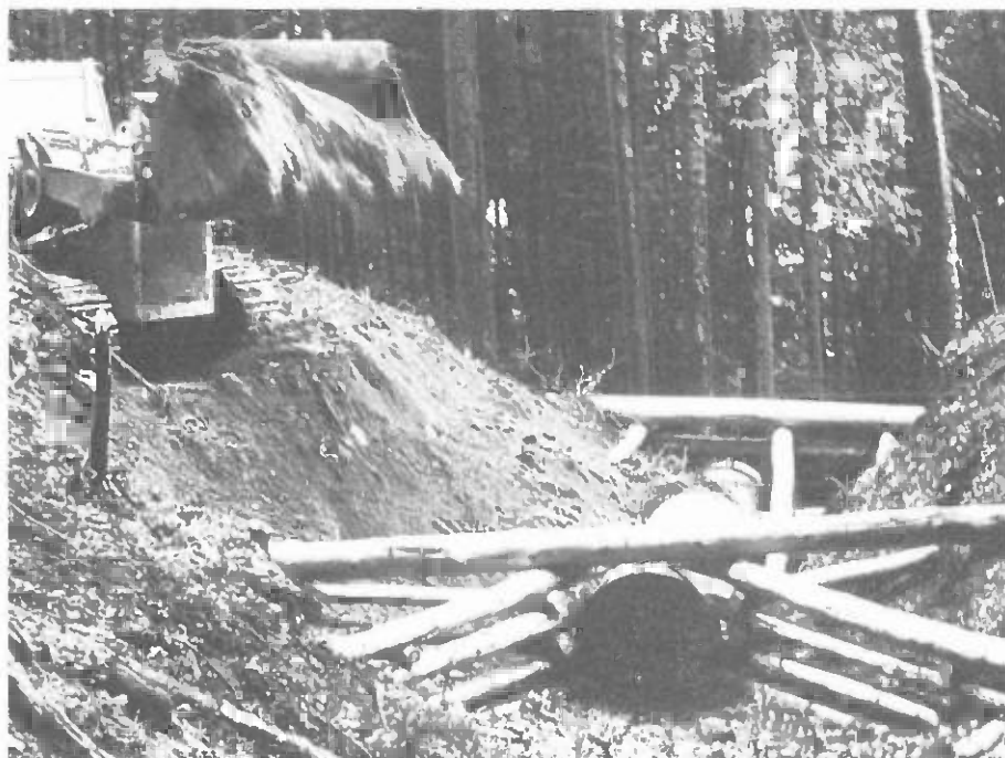
A gully being filled by traxcavator, concrete culvert and supporting roundwood construction laid so as to guarantee natural waterflow
