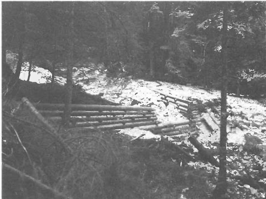
A series of check-dams made of roundwood at the top of a scree cone (Photo: M. Jedlitschka)
