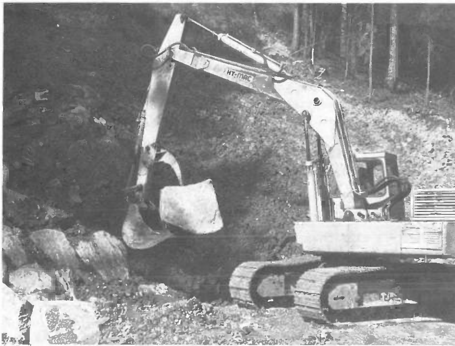
Construction of a retaining wall consisting of rock boulders placed into the cut slope by excavator (Photo: O. Sedlak)
