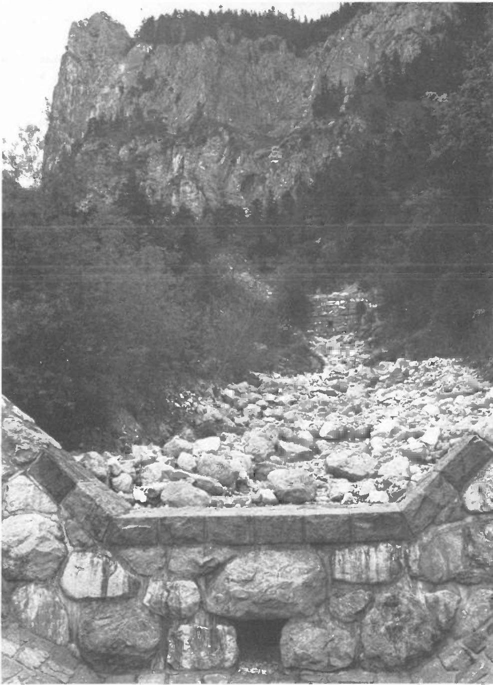
Sturdy rock-built check-dam in mountainous terrain in Austria
