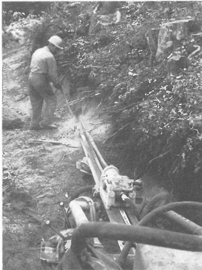
Tractor-mounted rock-drill used in mountain forest road construction (Photo: E. Pestal)
