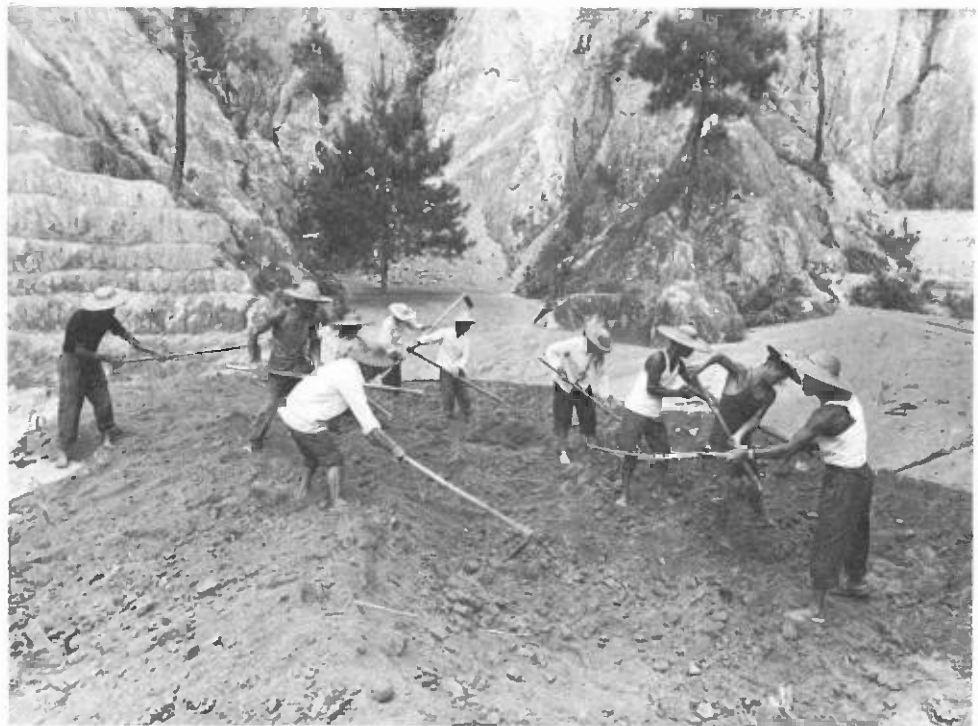
Erosion control. Making a check dam in Guangdong province to arrest silt
