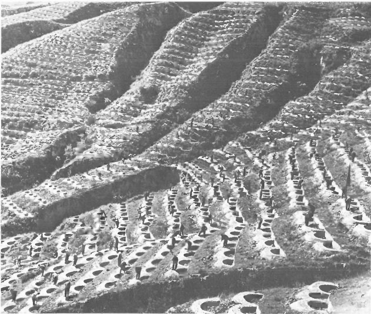
8-8: Terrace planting for erosion control in the loess region.
