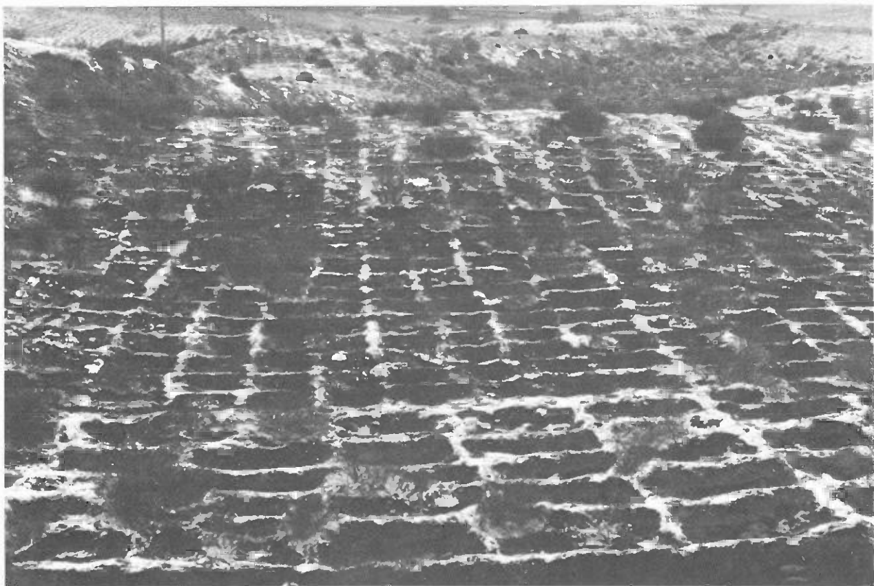
8-6: Sand dune stabilization project in Ninxia (Ningsia) Autonomous Region.
