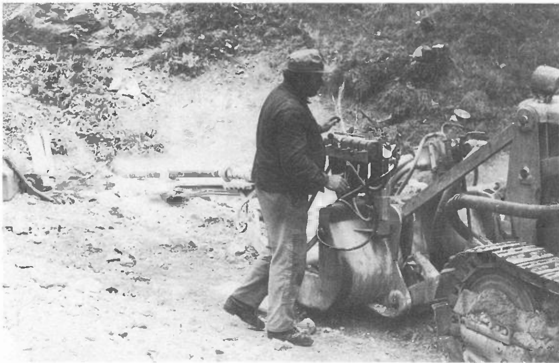
For larger rock volumes rock hammer drills mounted on tractors are often preferred (Photo E. Pestal)
