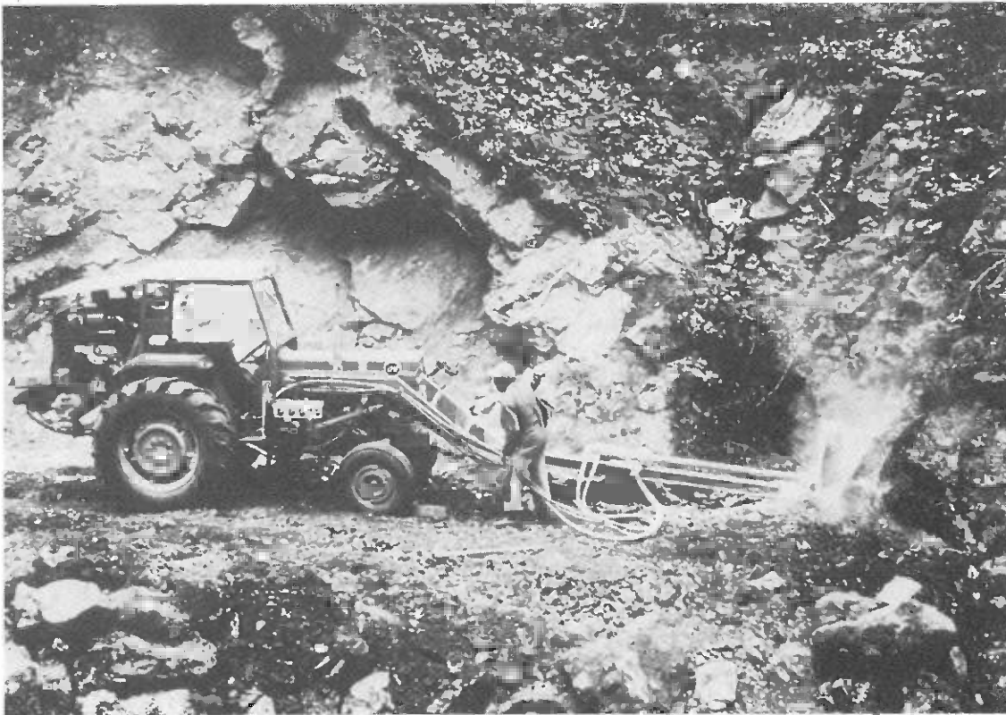
On dangerous construction sites, enterprises prefer to employ drills mounted on wheeled tractors because damage caused by falling rocks is cheaper to repair on these than on more costly crawler tractors. (Photo E. Pestal)
