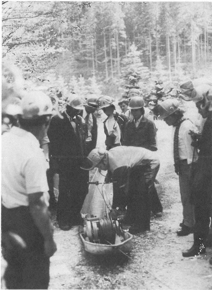
Sledge winch used in extraction of thinnings, and positioning of plastic chute (Photo R. Heinrich)
