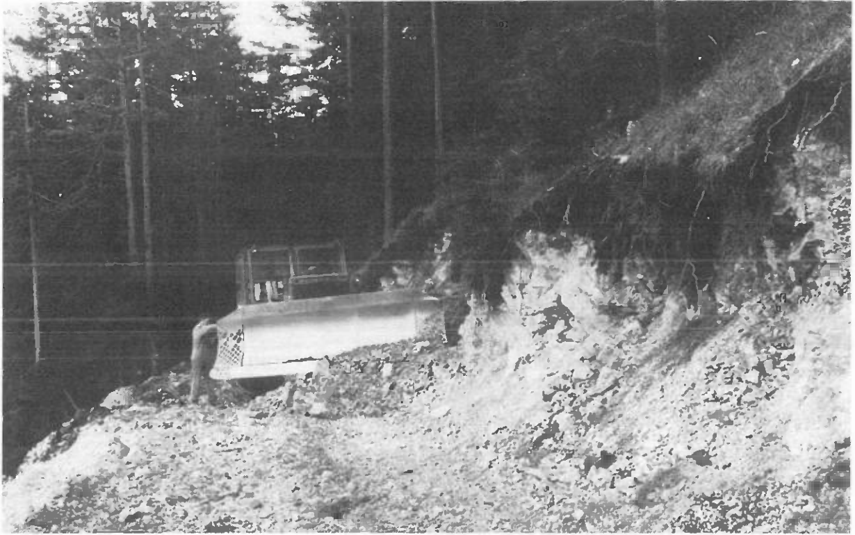
Angledozer excavating soft rock. (Photo E. Pestal)
