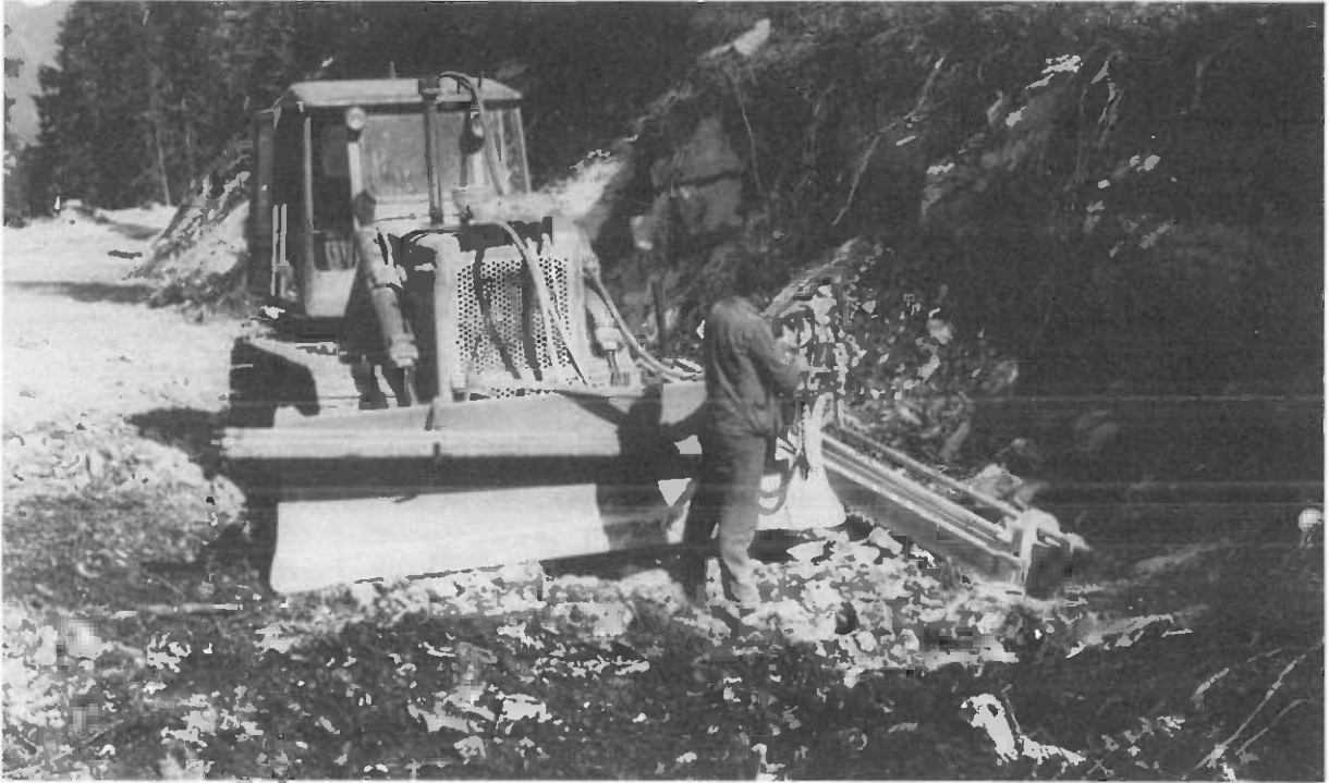
The revolving drill method was originally applied in mining. Except for granites and gneisses containing quartz, the method is the quickest and cheapest. (Photo E. Pestal)
