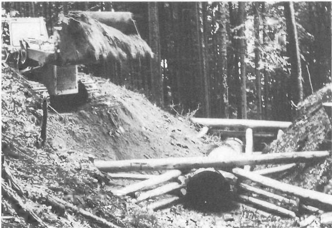
Fill of a gully by traxcavator, concrete culvert and supporting roundwood construction to guarantee natural waterflow. (Photo: FAO)
