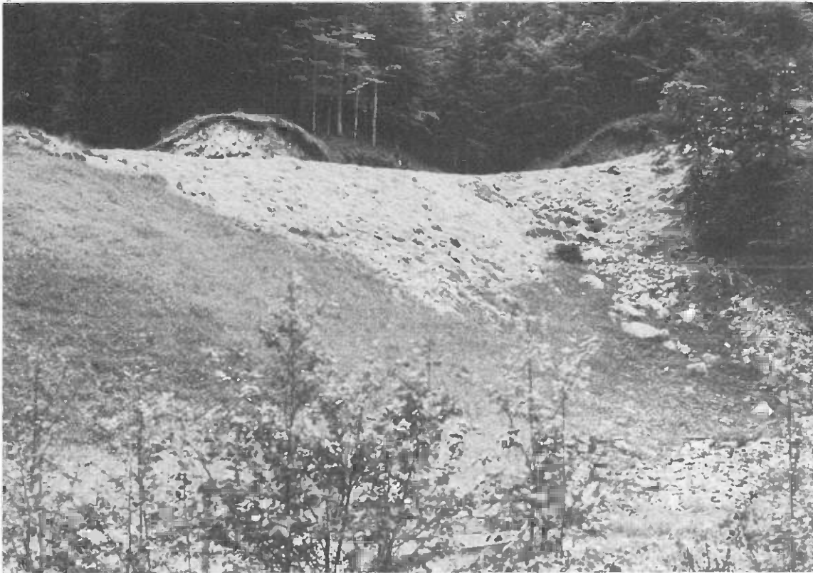
Revegetation of a fill slope by mulching (Photo FAO)
