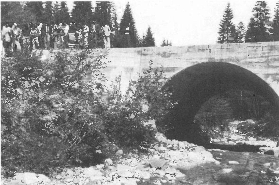
Corrugated steel sheet culvert used as form to replace a conventional bridge. (Photo T. Pasca)
