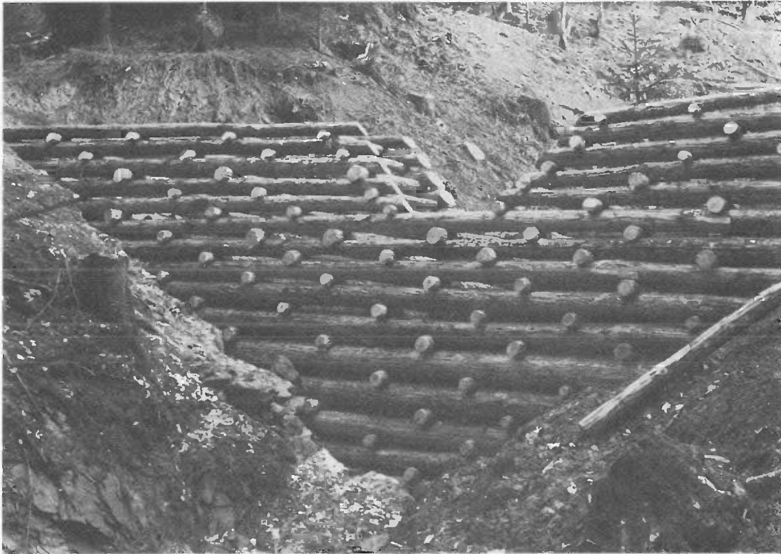
Crib type retaining wall made of roundwood to stop erosion by water flow. (Photo O. Sedlak)
