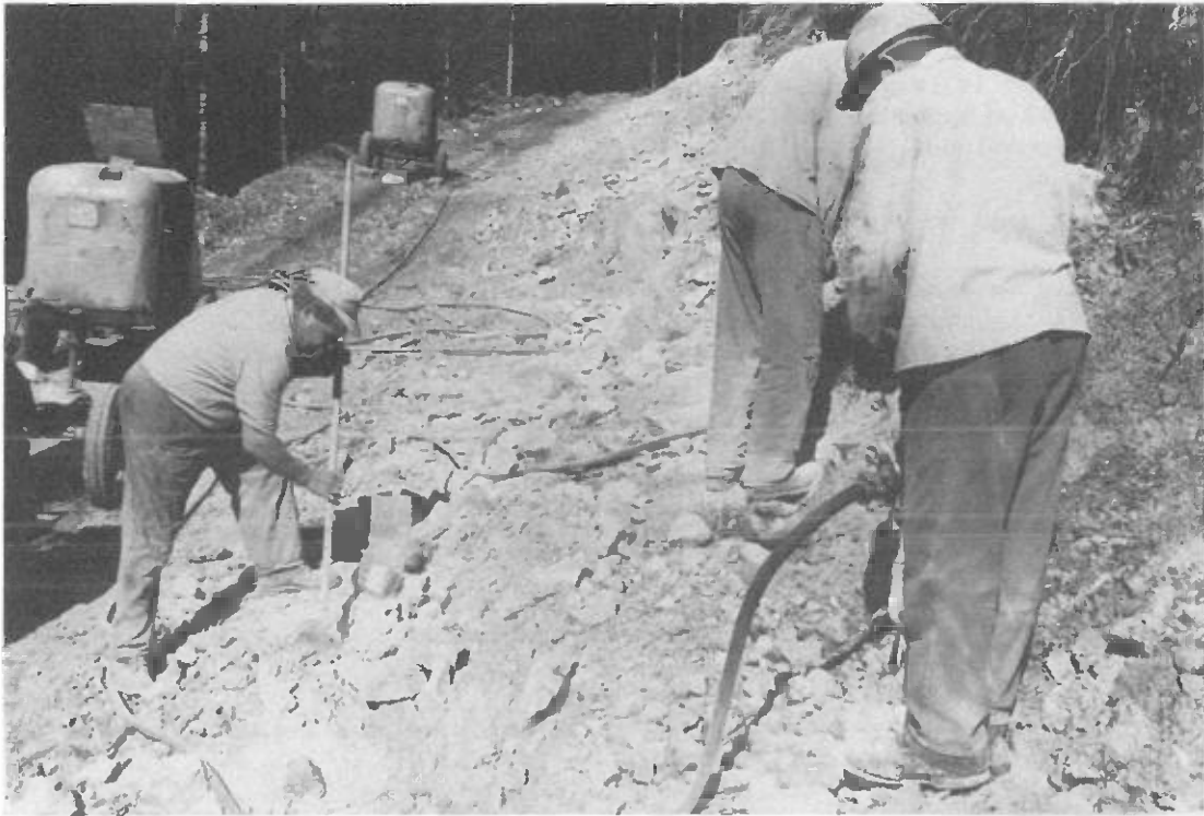
In areas with low volumes of rock or for final shaping and levelling, compressors and hand-operated rock drills are used in Austria (Photo E. Pestal)
