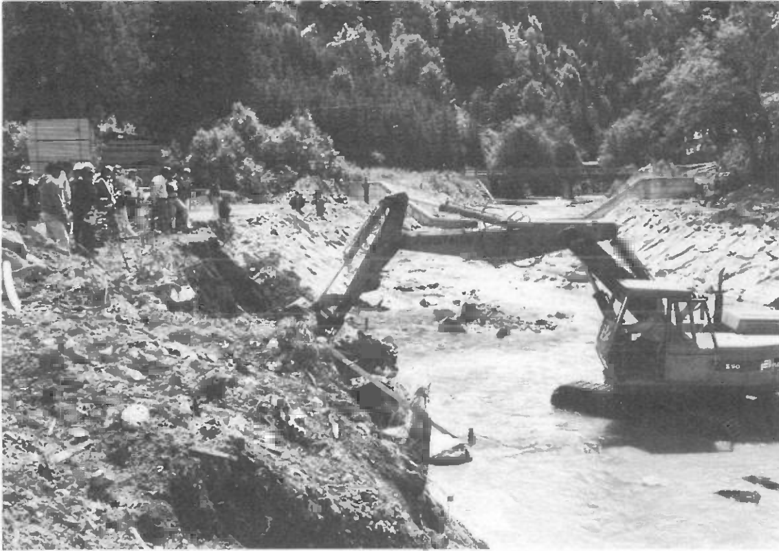
Construction of dry stone training wall to protect river banks. In the background, check dams protect bridge. (Photo T. Pasca)
