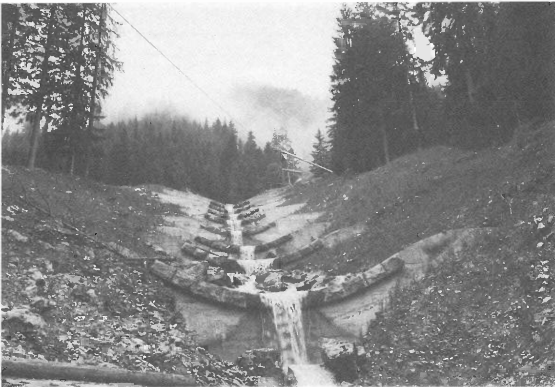
Torrent controlled with a series of check dams. (Photo T. Pasca)
