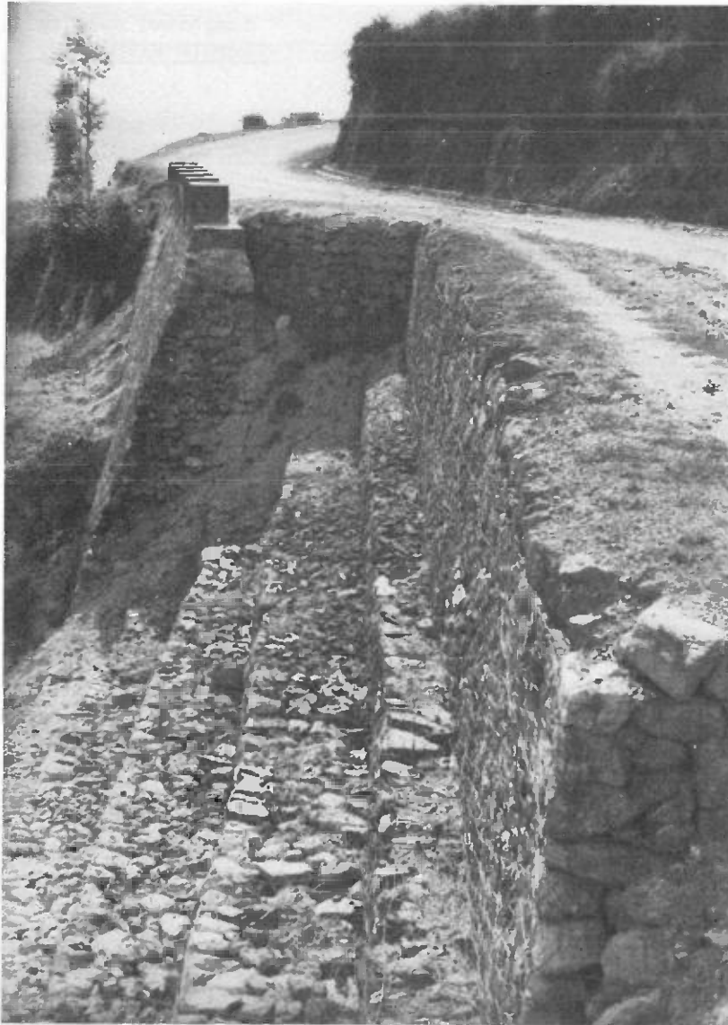
Roadbase and retaining wall destroyed by landslide; road fixed by gabion. (Nepal) (Photo FAO)
