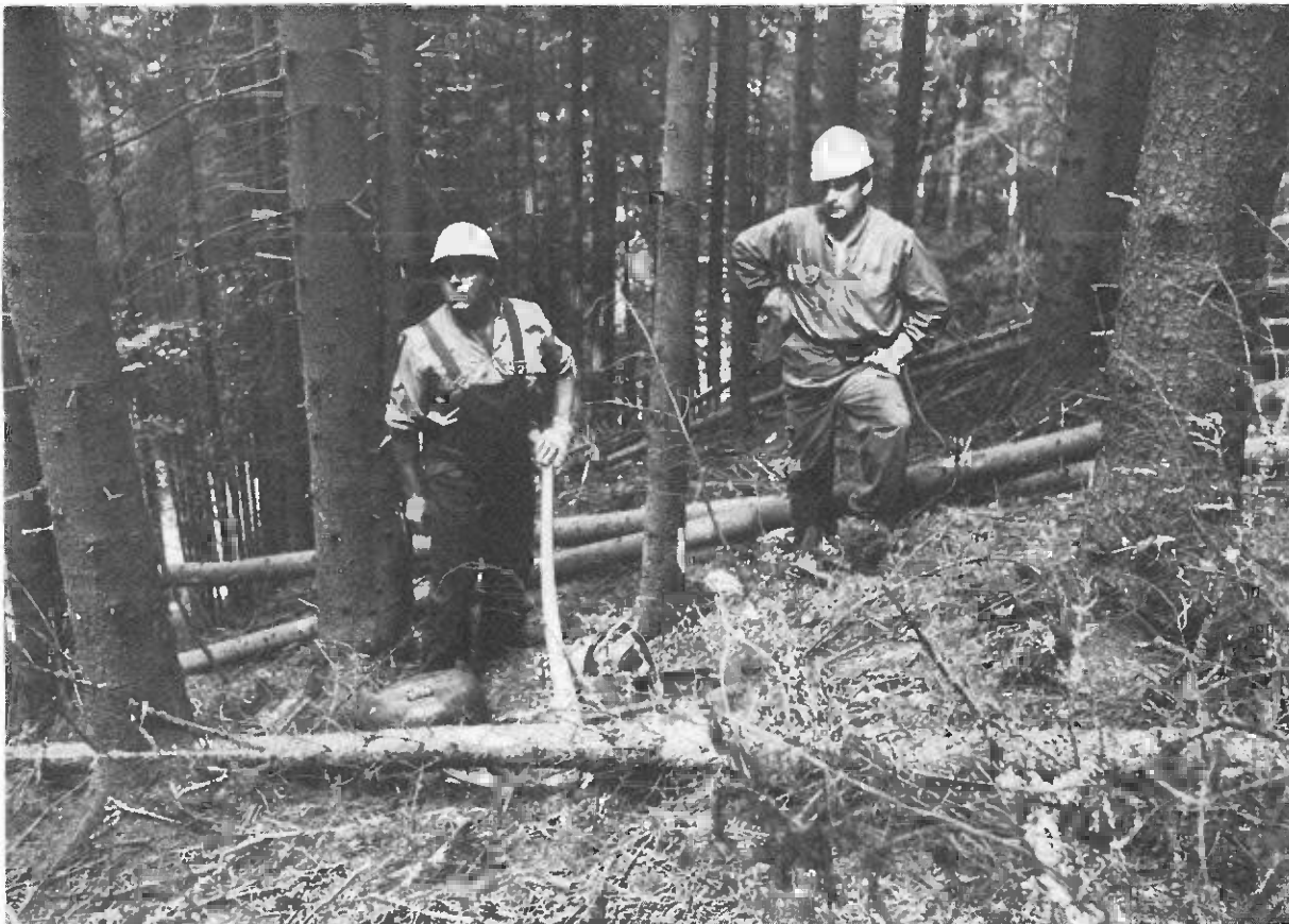
A pan used to pull down hang-ups when felling for thinnings. (Photo T. Pasca)
