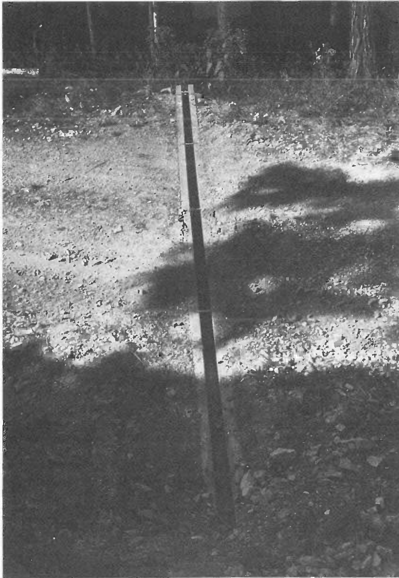
Wooden open top box culvert for road surface water drainage. (Photo: Federal Forestry Research Institute)
