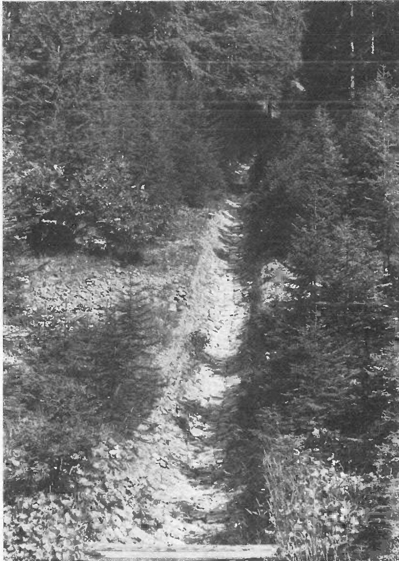
Water flow with pitched stones and revegetation cover on both sides of the water flow (Austria). (Photo FAO)
