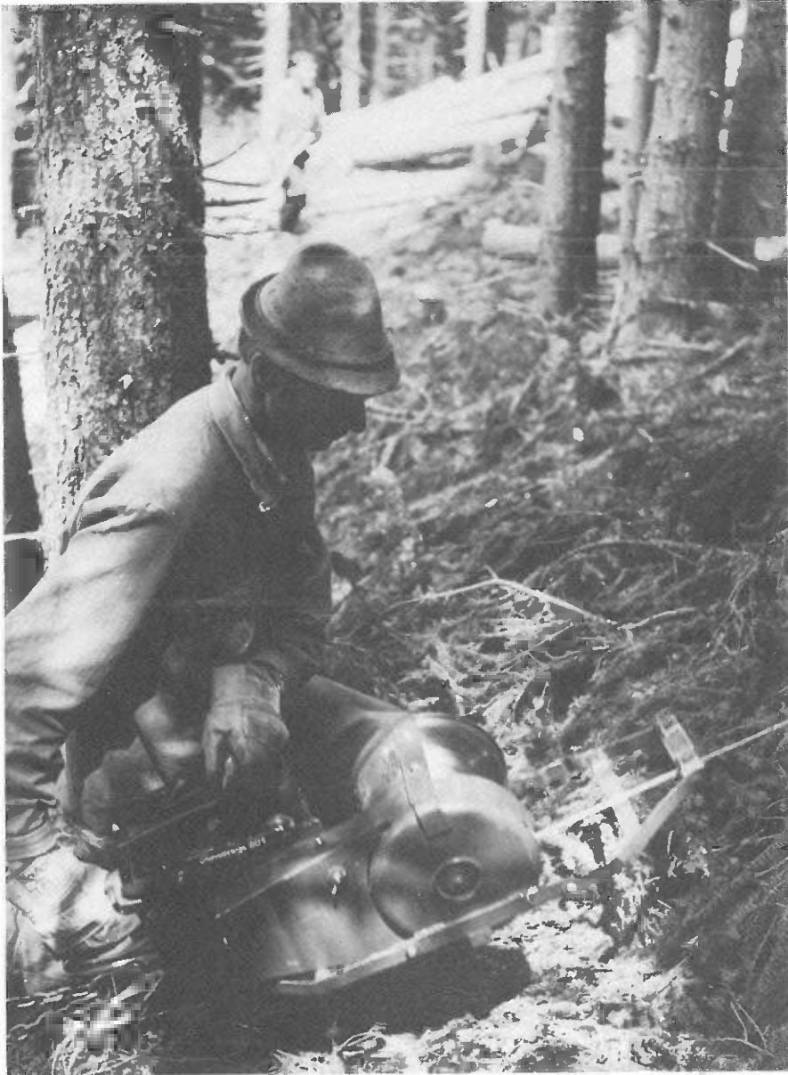
Power saw winches are useful when clearing forest roads. (Photo E. Pestal)
