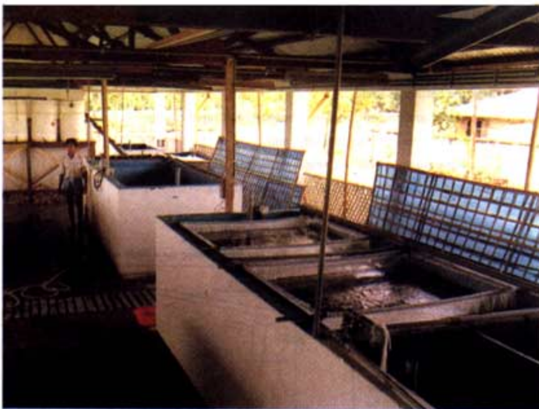
Ag. 5 Interior of small-scale freshwater prawn hatchery. Larval rearing tanks in the foreground, brine storage and mixing tanks and sand filters in background
