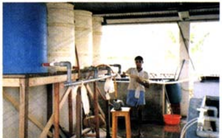
Fig. 7b 200 l plastic barrels converted to rapid sand filters
