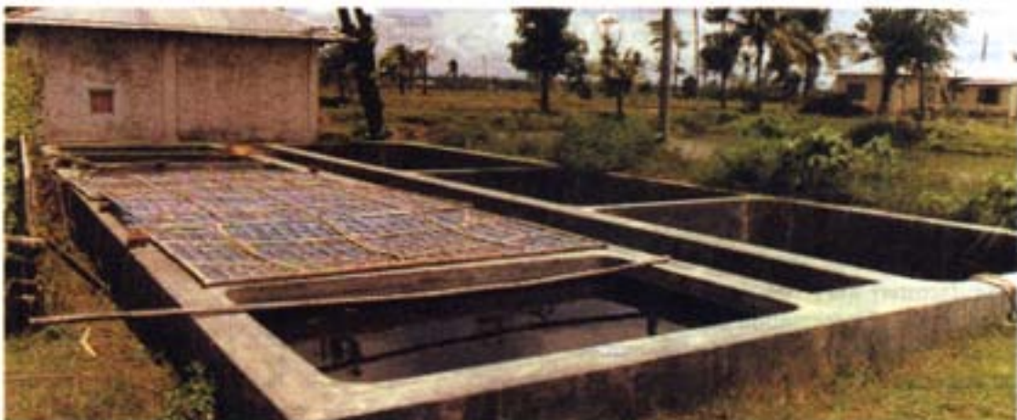
Fig. 10 Plastered brick outdoor holding tanks for broodstock, berried females and post-larvae.
