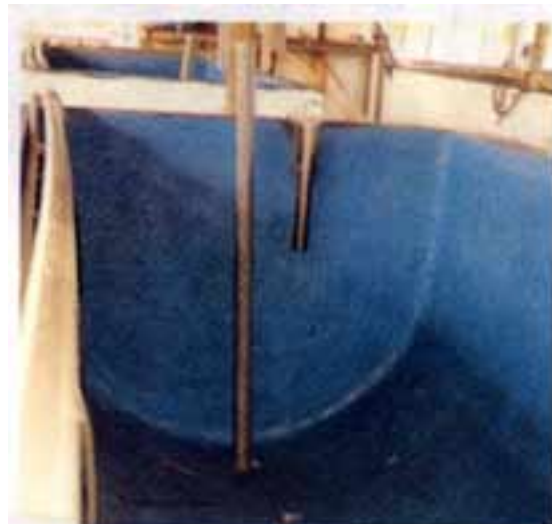
Fig. 12 Round bottom, 5 t larval rearing tank showing interior epoxy coating, stand pipe drain and 2 kva immersion heater
