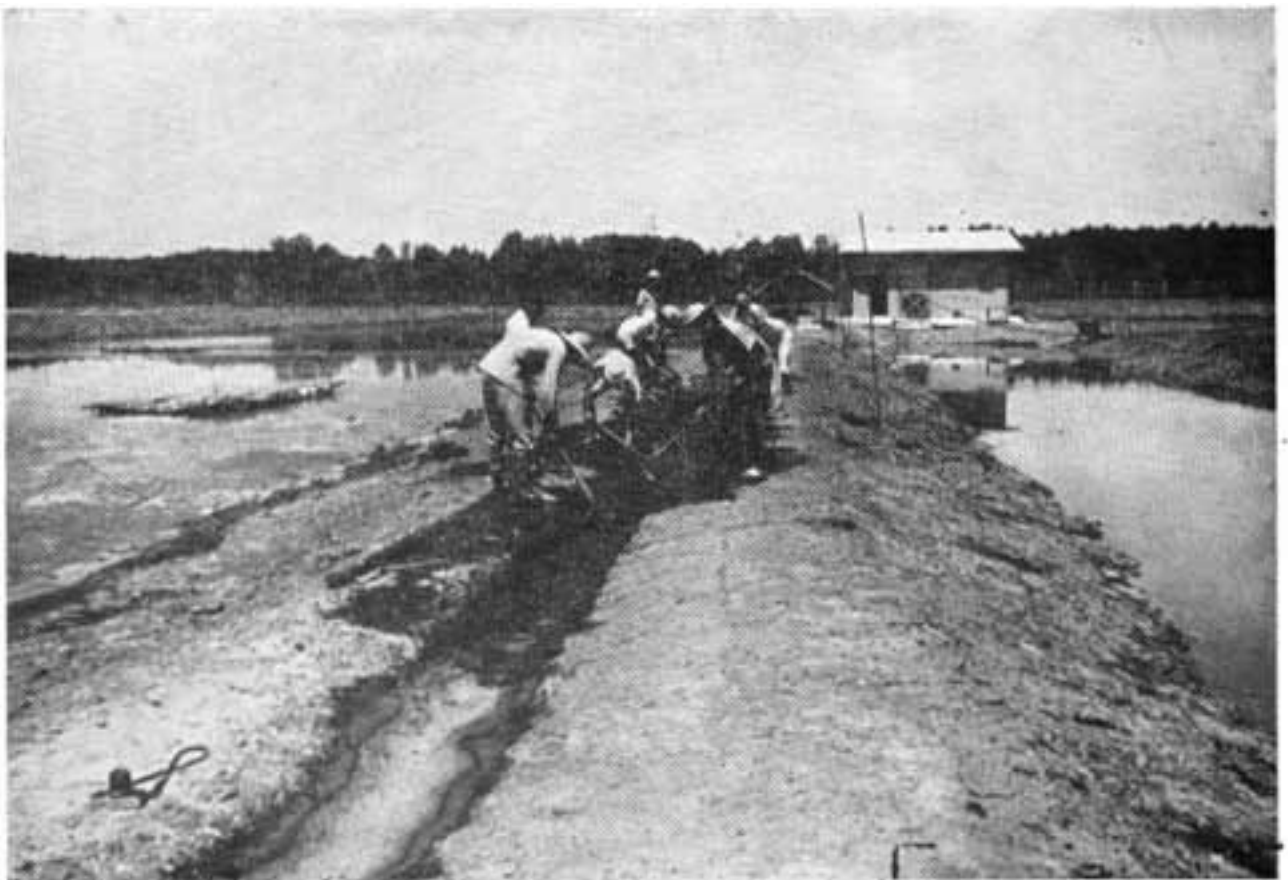
Digging of dyke trench is in progress—a prelude to water and lime treatment.
