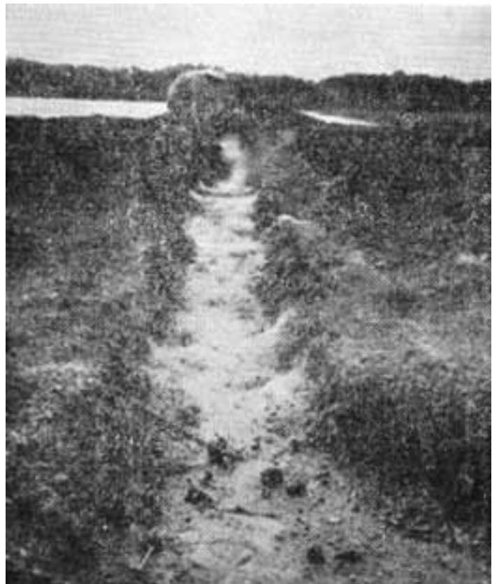
Applying lime to the soil dyke to reduce acid sulphate content of the soil.
