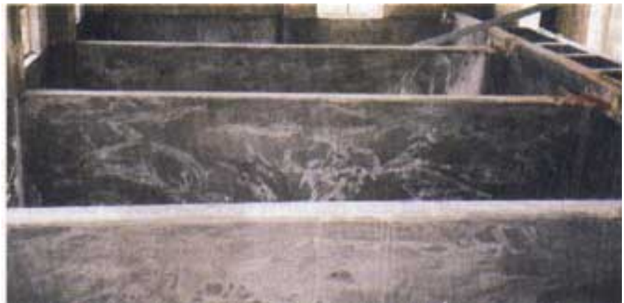
Crescent Fish Farms under construction, Jhodipur, Bangladesh.
