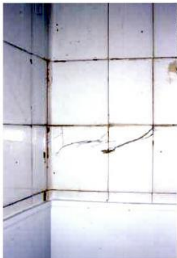
PHOTO 10.4 Avoid: cracked tiles: they can provide a refuge for micro-organisms
