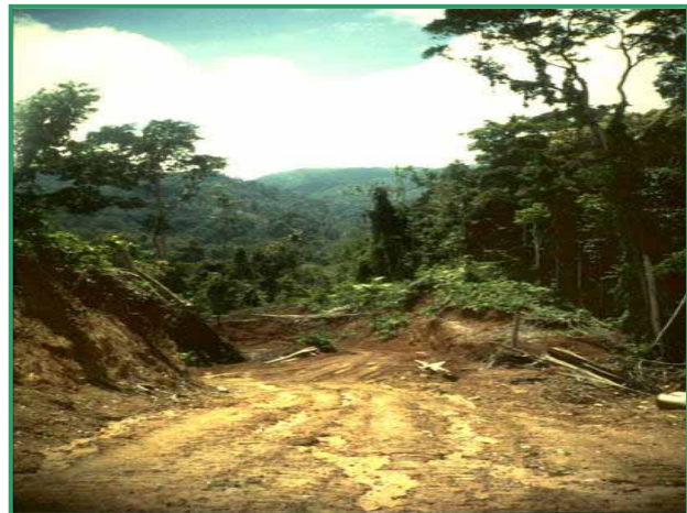
Erosion caused by poor road construction
