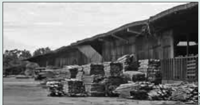
A mill site in Indonesia
