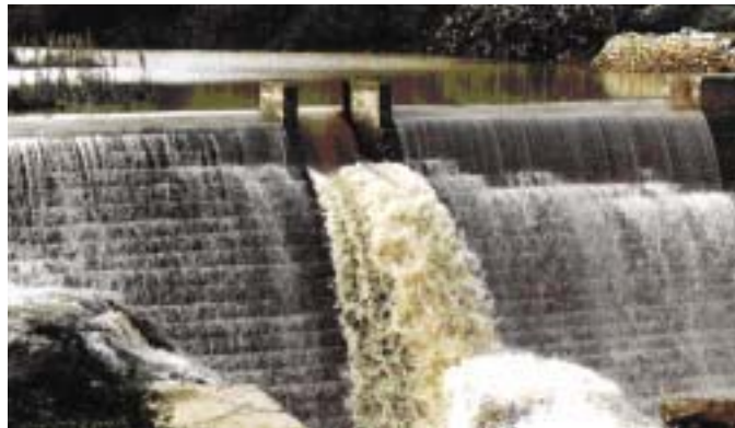
Plate 5 Dam at Wied is-Sewda.
