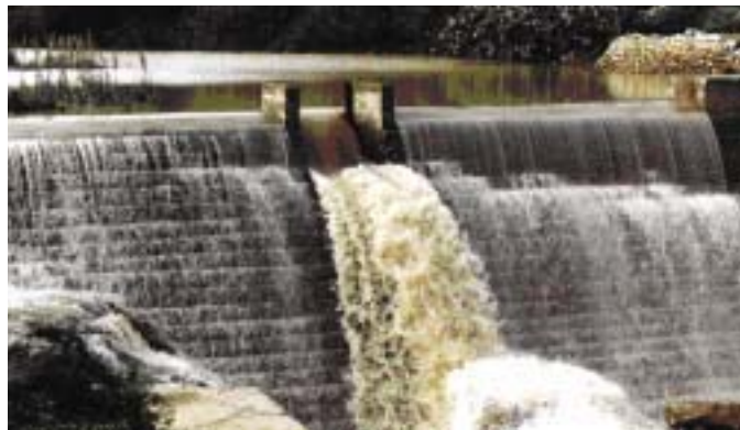
Plate 5 Dam at Wied is-Sewda.
