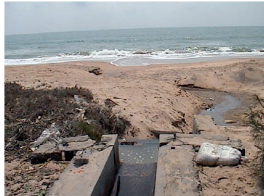
Effluent discharge into the open sea adjacent to a hatchery without any treatment increases risks of disease
