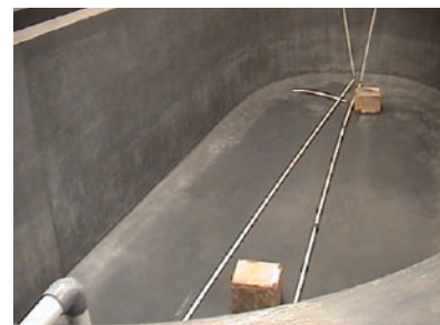
Larval-rearing tanks at some hatcheries are not painted with epoxy so cleaning is difficult
