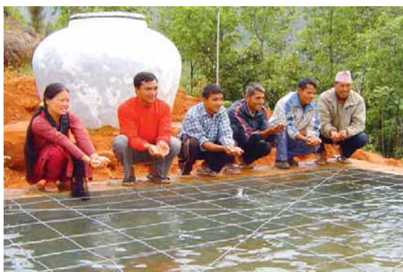
Combination of Thai Jar and underground water tank in a MUS, Nepal.
