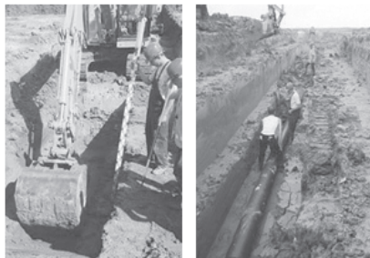
FIGURE 17.2 - Installation of the pipes.
