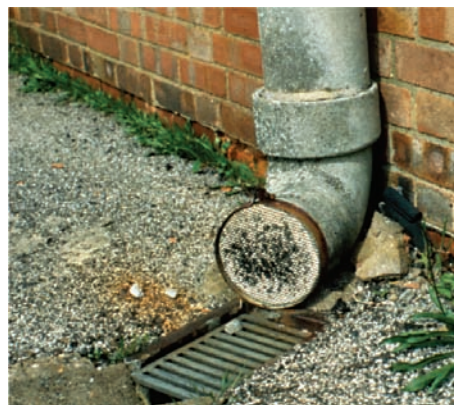
FIGURE 23 Screening a drain pipe to prevent rodent entry
