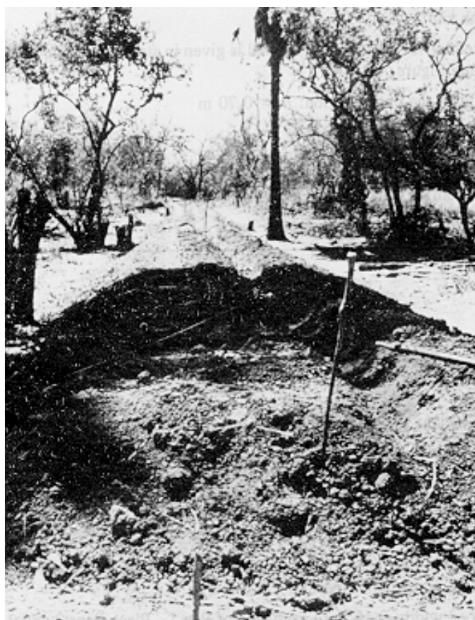
FIGURE A2.8 Embankment under construction
