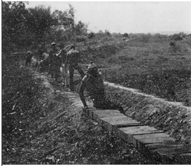
FIGURE A2.4 Canal in fill
