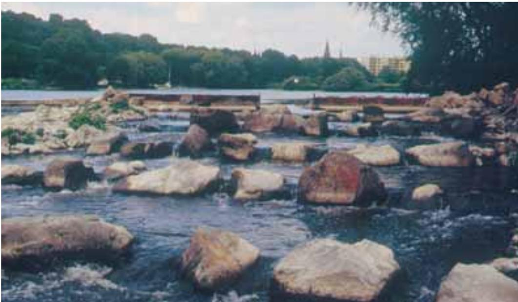
**Figure 4.41:** Spillenburg weir; fish ramp after completion
