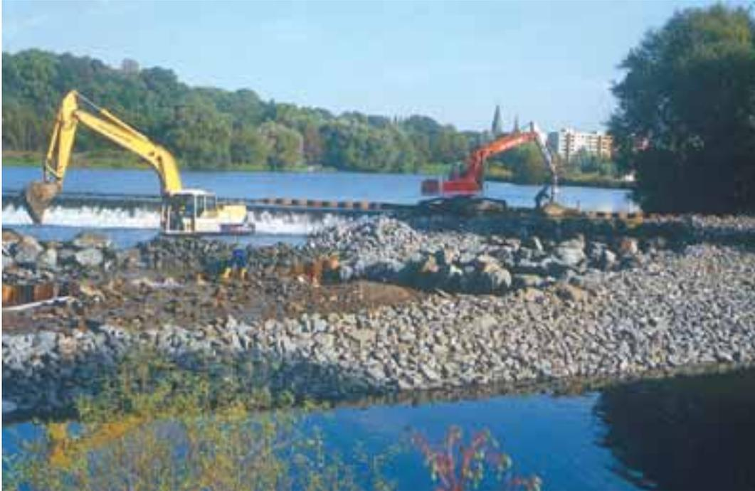
**Figure 4.40:** Spillenburg weir; fish ramp under construction
