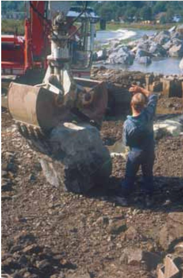
Figure 4.38: Setting the boulder bars
