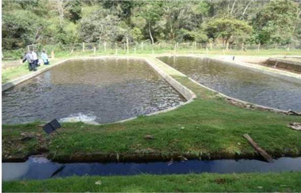
Figure 4: Concrete Trout raceways
