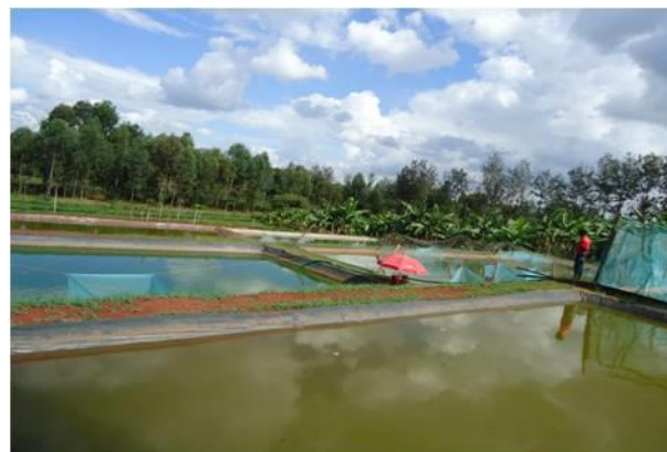
Figure 3: Earthen pond and Lined ponds in aqua farms in Kenya
