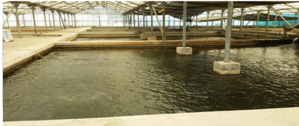
室内池塘Indoor concrete pond
