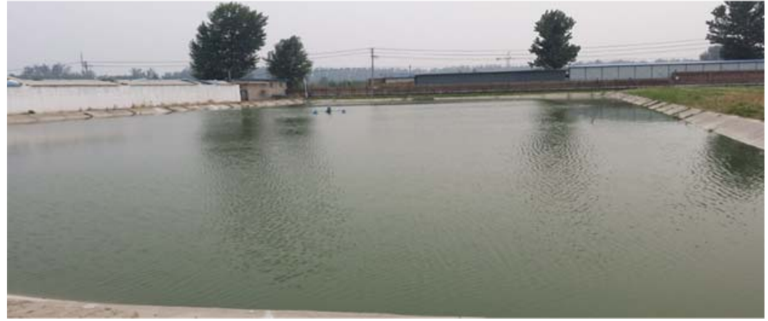
水泥护坡的池塘Pond with concrete slopes
