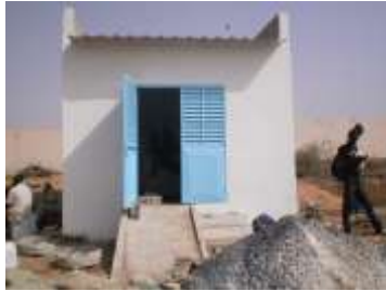
Shelter for power driven pump
