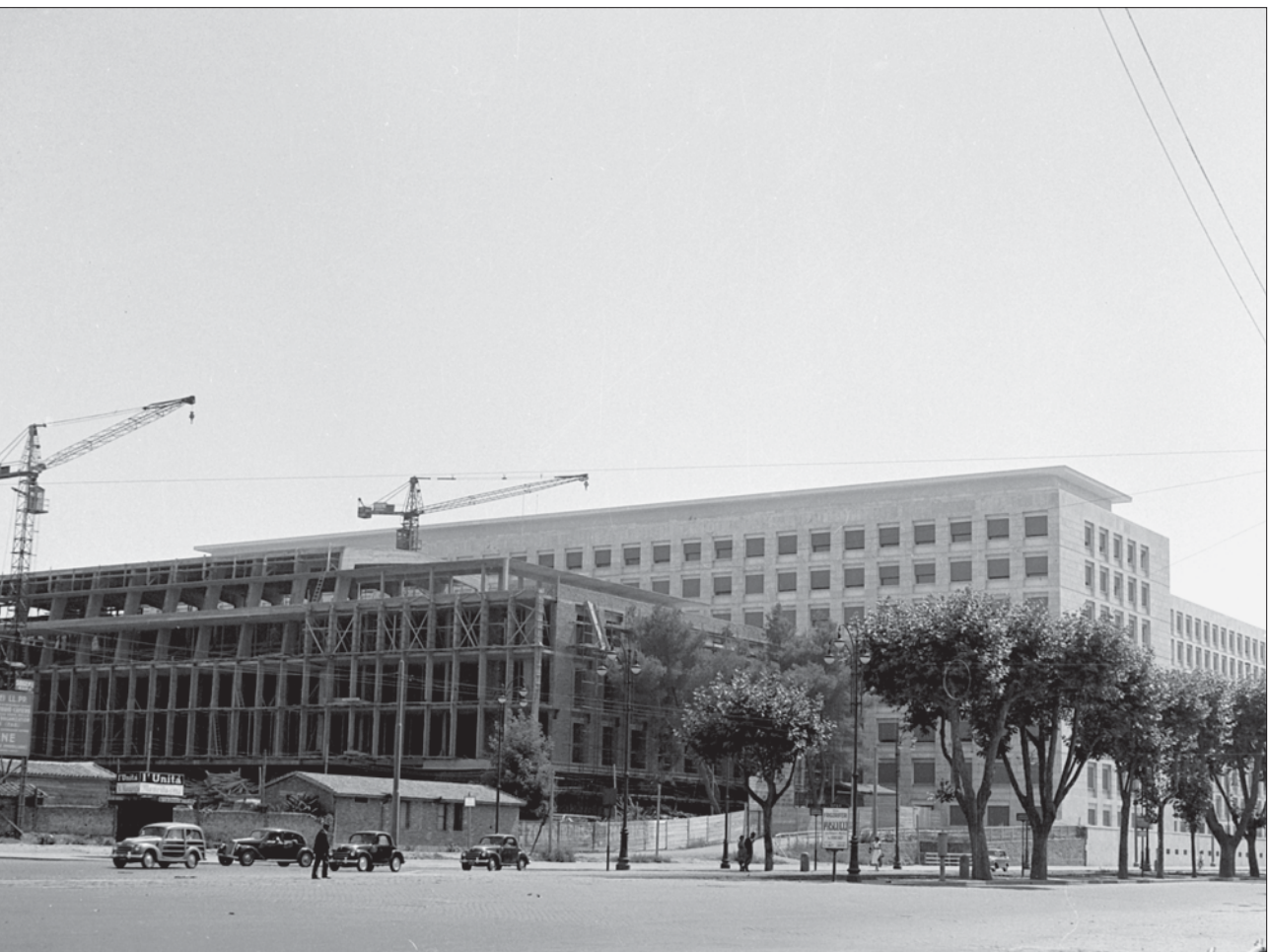
Rome, 1951: works under way on one of the buildings that will host FAO.
