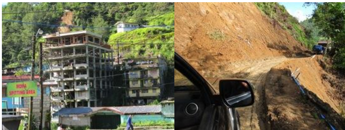
Figure...Constructions lies incomplete due to the lack of financial capital in Banawe the center of Iugao tourism. (left) Landslides happen quite often everywhere in Ifugao because of deforestation that also hinders transportation services (Right).
