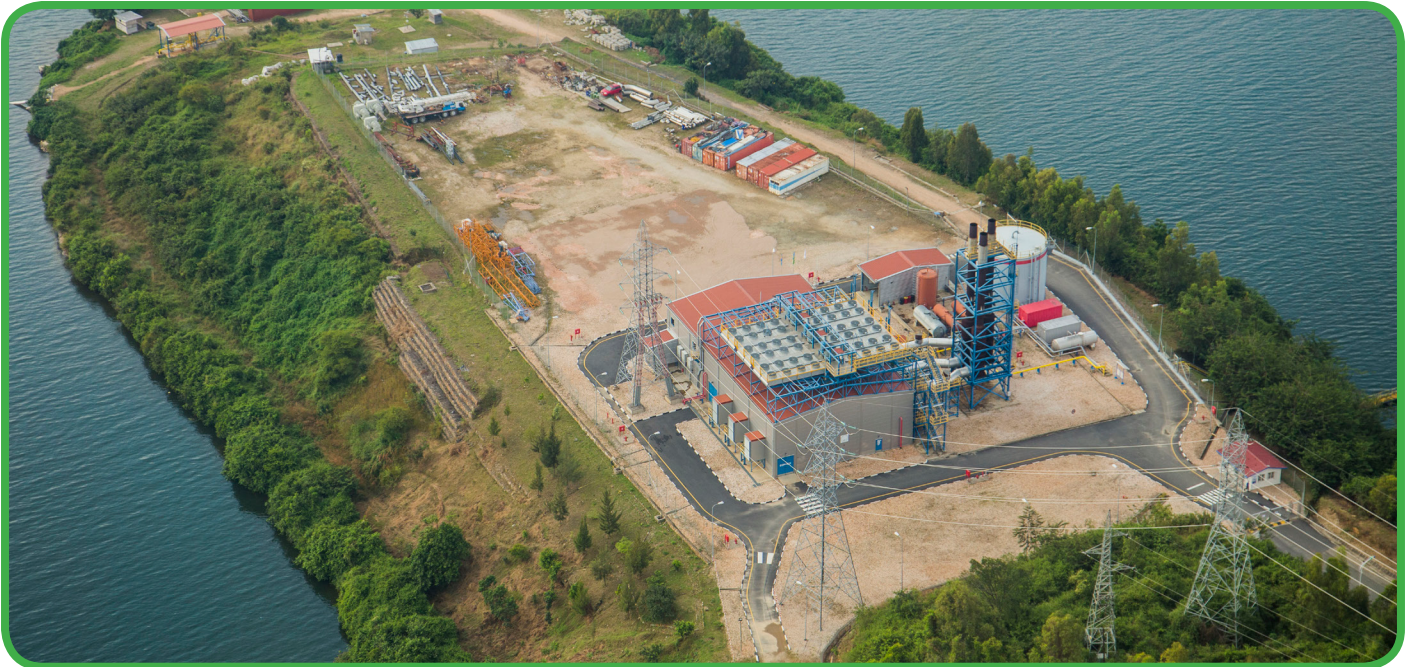
Rwanda started producing electricity from methane gas pumped from Kivu. Kivu watt production plant. Photo by Cyril N.
