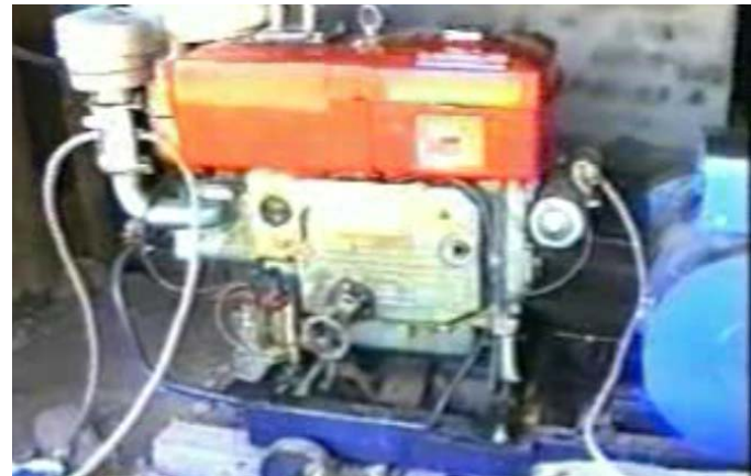
Generator utilizing biogas
