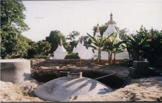
Almost completed biogas tank in a village
