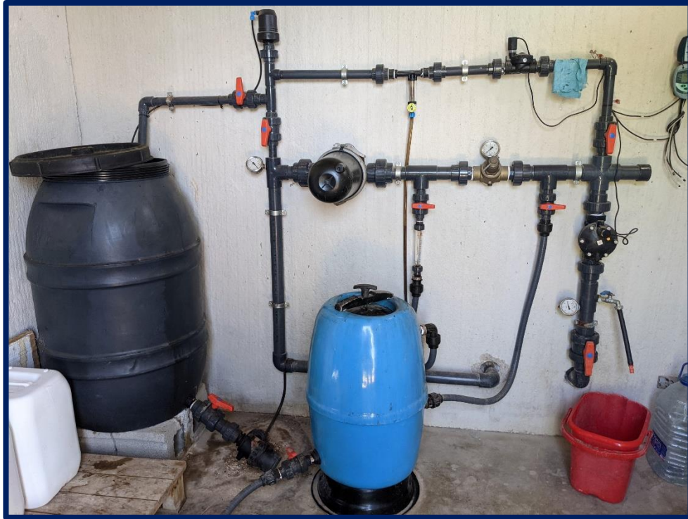
Drip ferti-irrigation system (Copyright: Simeón Ruíz Cayuela)
