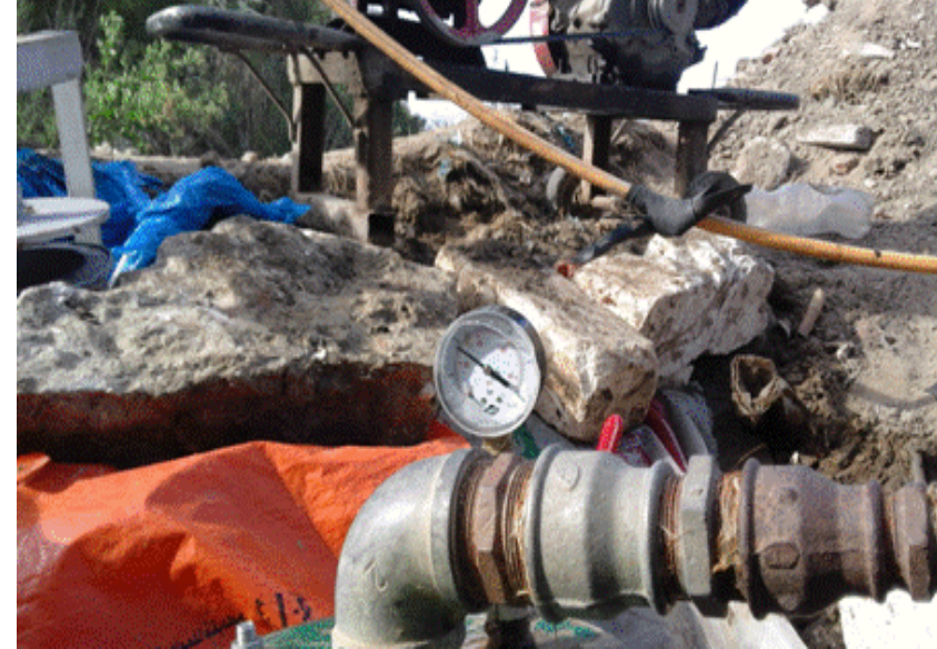
After 30 minutes measured pressure 1.9 bar.
