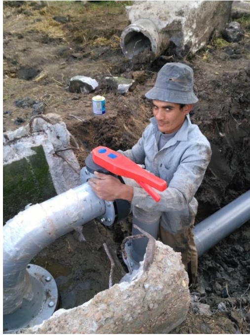
Installation of Butterfly Value works
