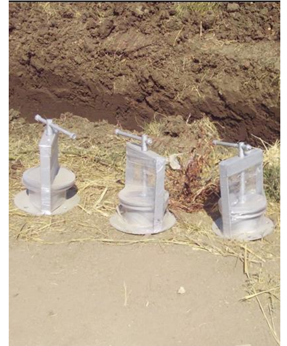
Hydrant Valves to be installed
