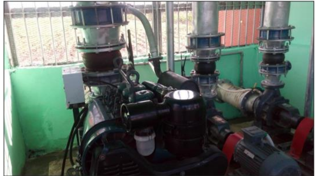
Installation of 2 electrical Units and Diesel Unit
