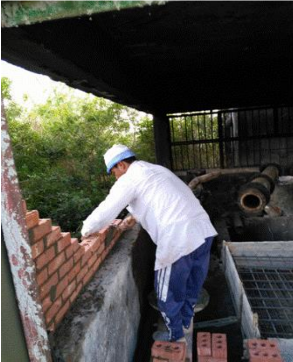
Brick Works for Pump Room
