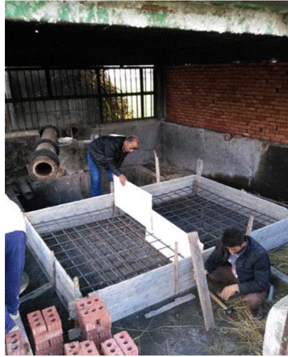
Foundation Works for Electrical & Diesel Pumps
