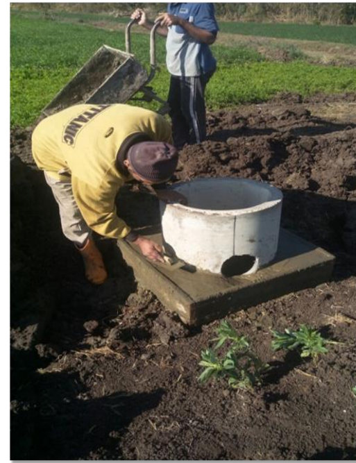
Concrete Foundation for Hydrant Concrete Protection
