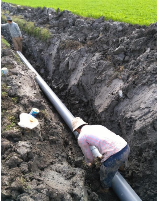
Laying UPVC Pipe Works
