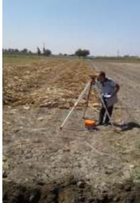
Survey works for checking the excavation level under pipes.
