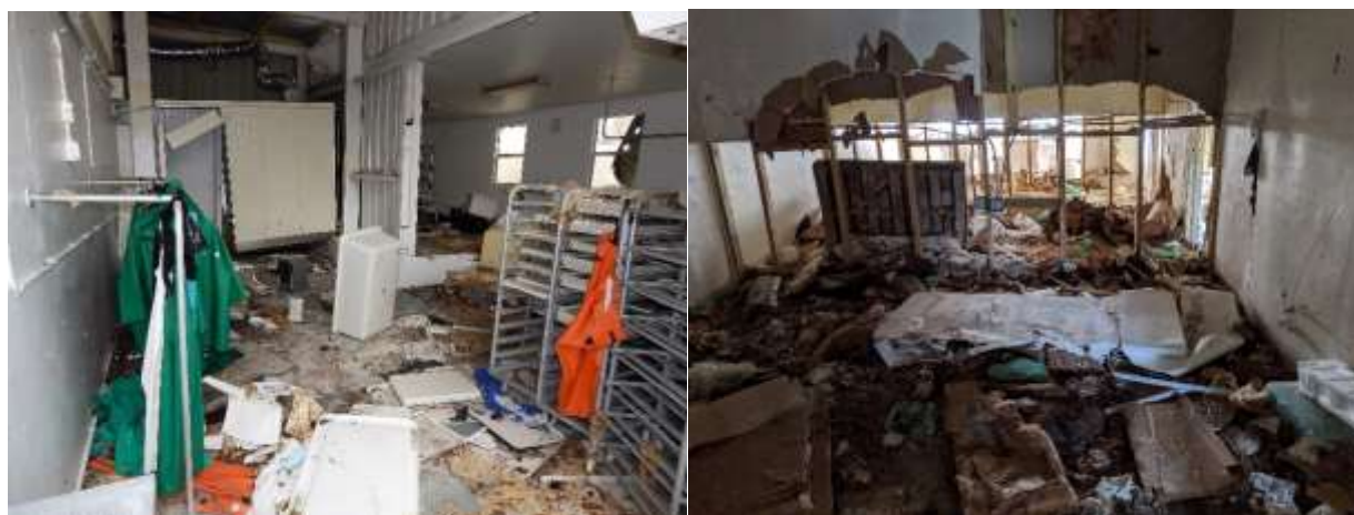
Figure 9. Inside two processing plants shortly after the flood: left-hand side picture shows a plant in Marsh Harbour, and the righthand side picture shows a packing area inside a processing plant in Freeport (authors).
