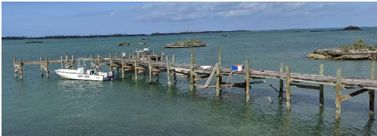
Figure 8. A typical wooden jetty in The Bahamas. The wooden deck was removed before the hurricane passed and put back on after (authors).
