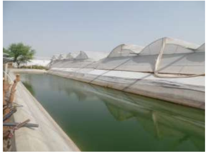
Figure 2. Ponds for rainwater harvesting.
