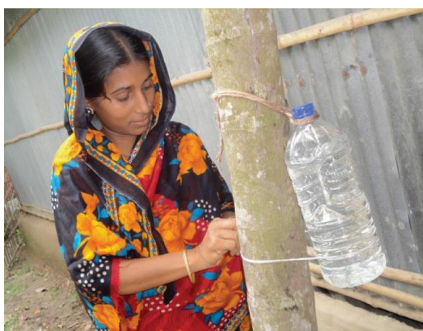
Fig. Installing a tippy tap on a tree Source: SPRING promotion materials – How to Build Your own Tippy Tap
