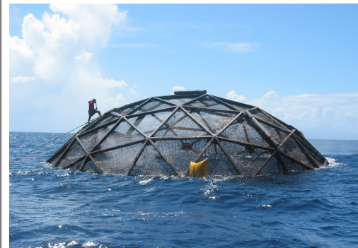
Aquapod – geodesic sphere, submersible
