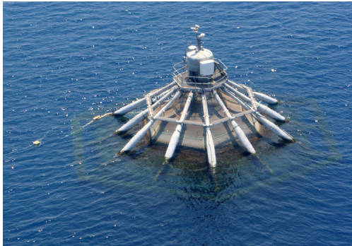
FarmOcean cage – semi-submersible, reduced surface exposure
