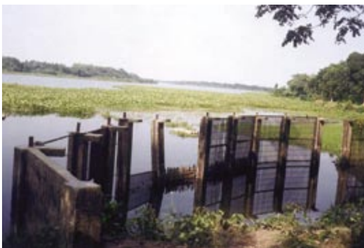
An oxbow lake with partially broken metallic screen in the outlet, Jessore, Bangladesh
