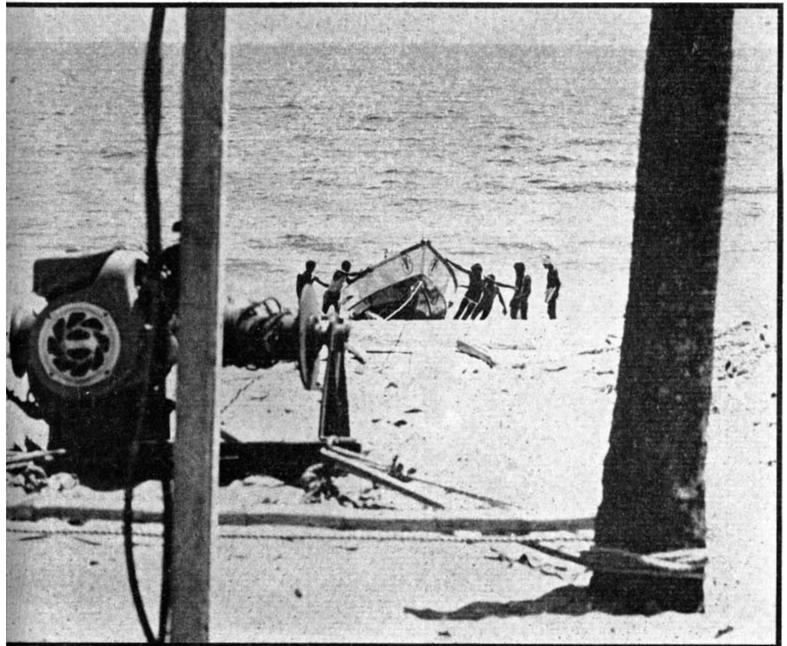
Above : The IND-20, a 28-foot beachlanding boat developed for Andhra Pradesh, is being launched using pneumatic jenders as beach rollers. Below: The boat is being hauled up the beach at liTjambakkam near Madras by a diesel-powered winch secured to palm trees. The winch has proved popular with fishermen.
