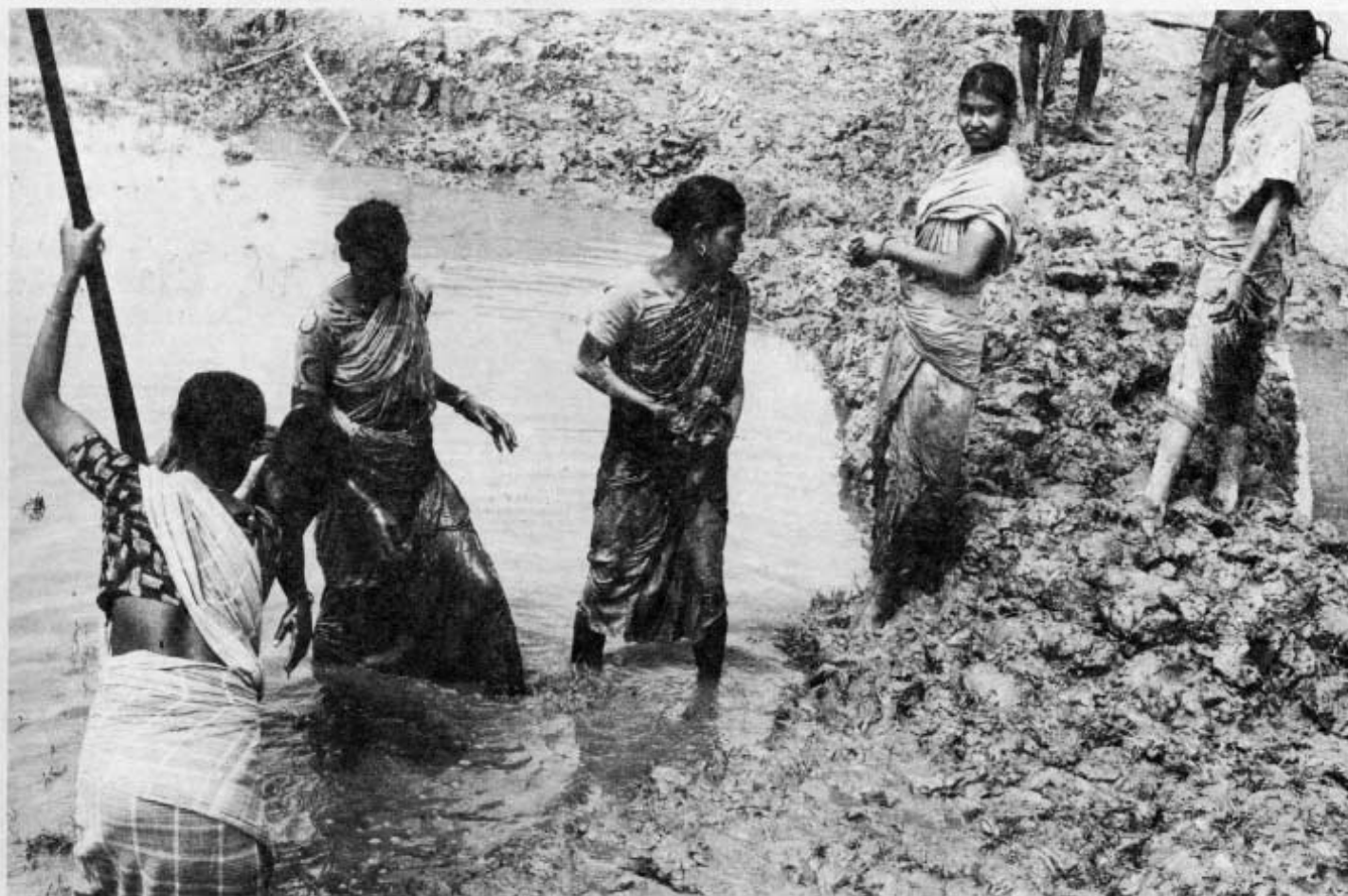
Repair of pond dyke by women construction workers at Satkhira.
