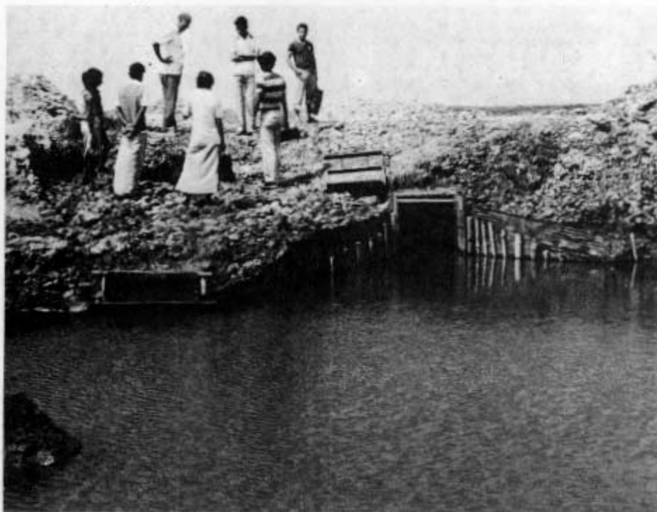
Project staff supervise maintenance work on the main sluice.
