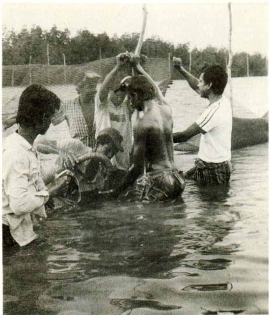
At the shrimp pen site in Chilaw, Sri Lanka, local fishermen are constructing Netlon pen walls. A water jet facilitates insertion of the pen wall into the lagoon floor.
