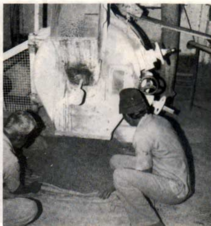
Left : Sieving of powdered feed ingredients to remove foreign matter and ensure fineness so that the feed is water-stable. Right : Shrimp feed comes out in pellets from pelleting machine.
