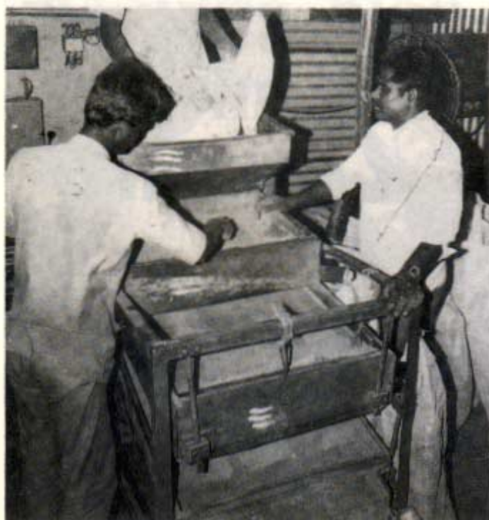
Left : Sieving of powdered feed ingredients to remove foreign matter and ensure fineness so that the feed is water-stable. Right : Shrimp feed comes out in pellets from pelleting machine.
