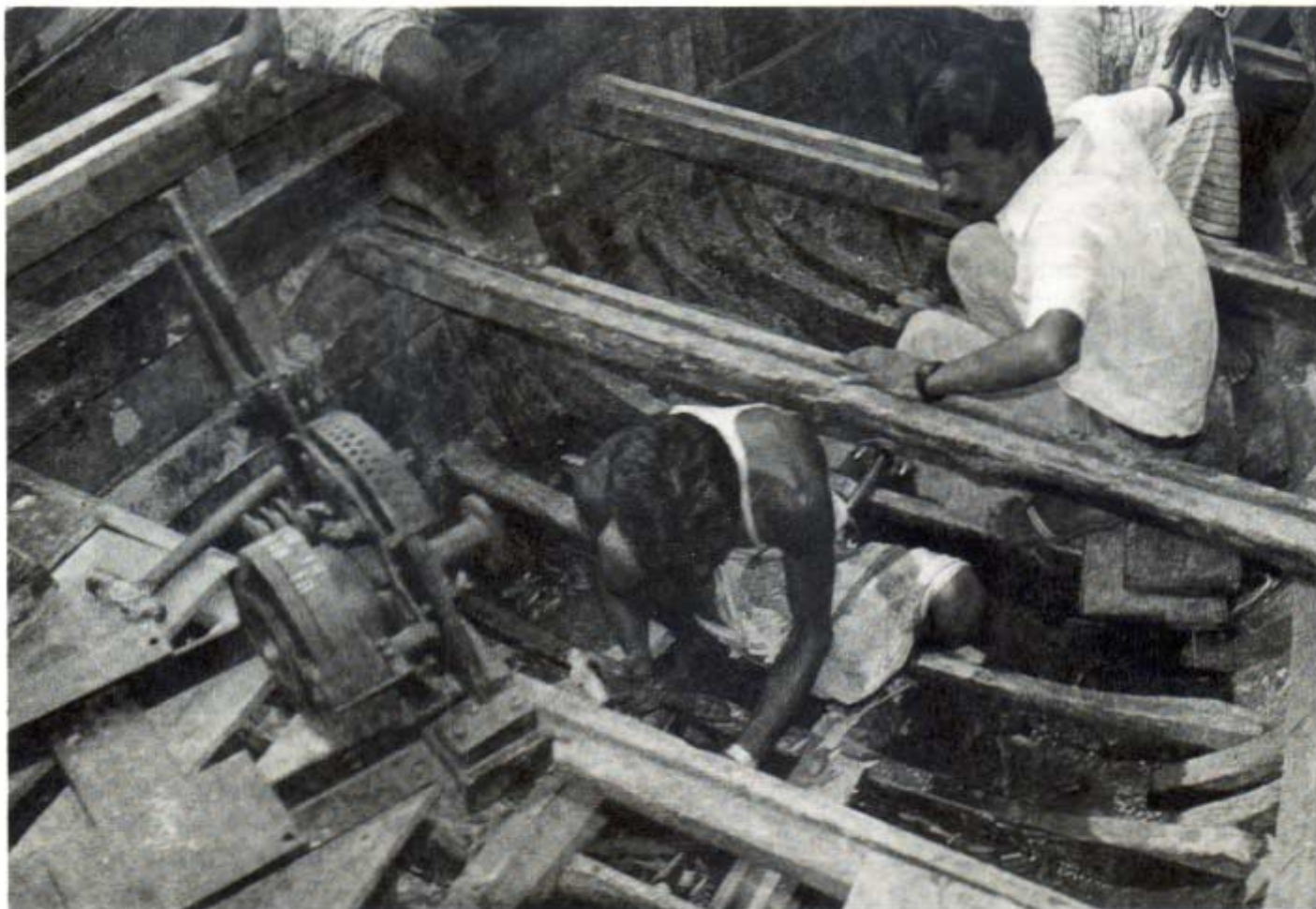
Installing an engine in a chandi boat.
