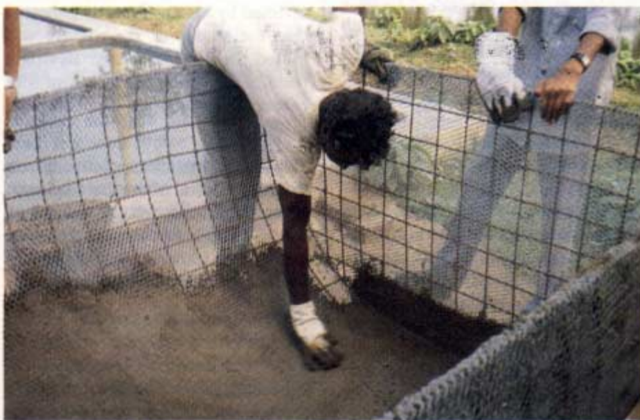
Plastering a ferro-cement larval rearing tank.
