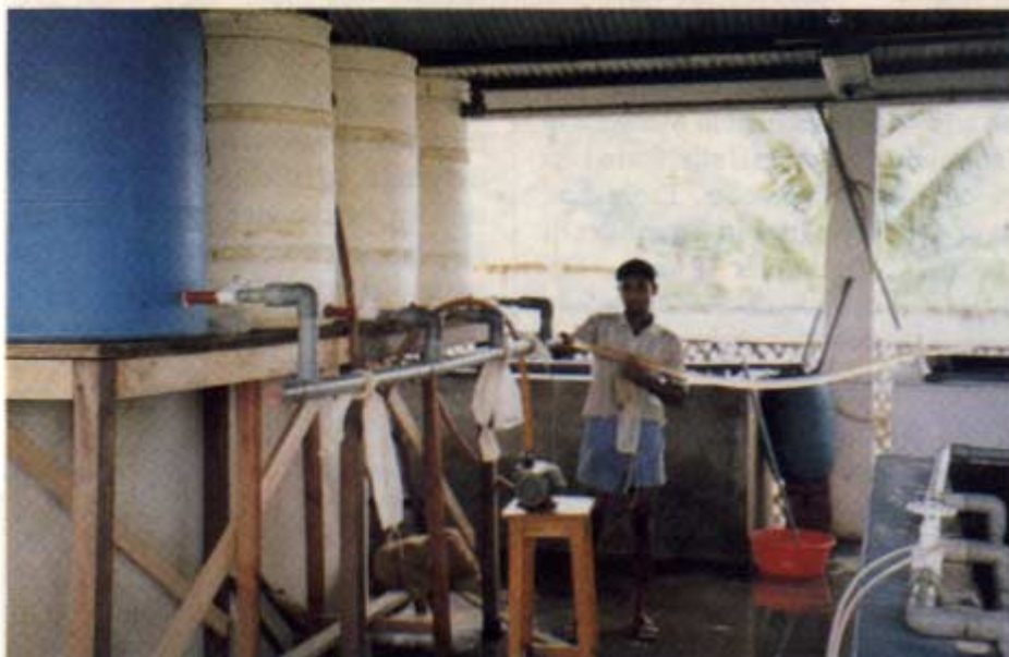
Sand filters used to filter rearing water after chlorine treatment
