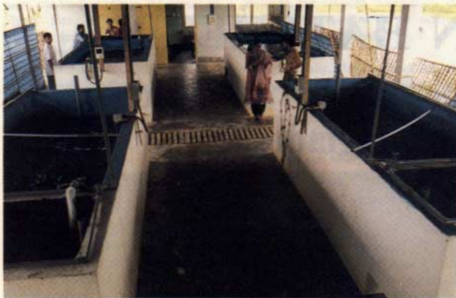
Sand filters used to filter rearing water after chlorine treatment
