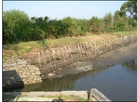
Figure 5 Different ways to enforce dyke against erosion
